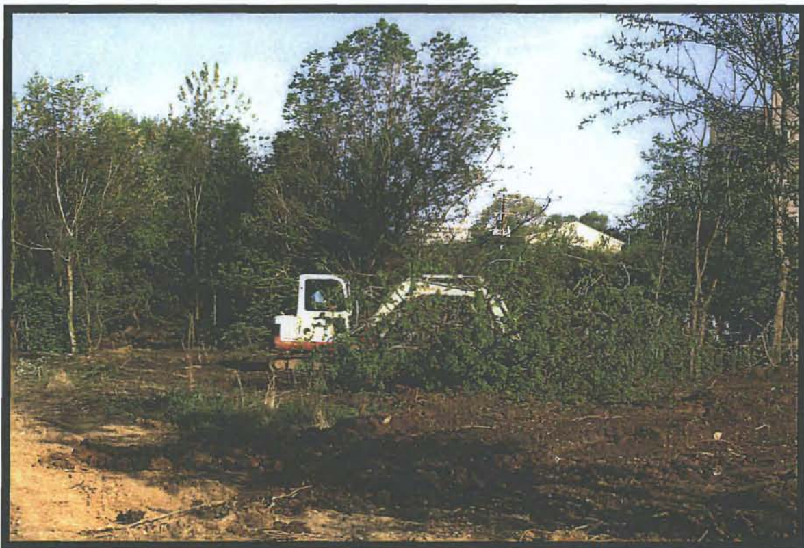
Plate 5.1 Western Overview of Project Area, Showing Backhoe Clearing Vegetation and Preparing Surface for Trench Excavations.
