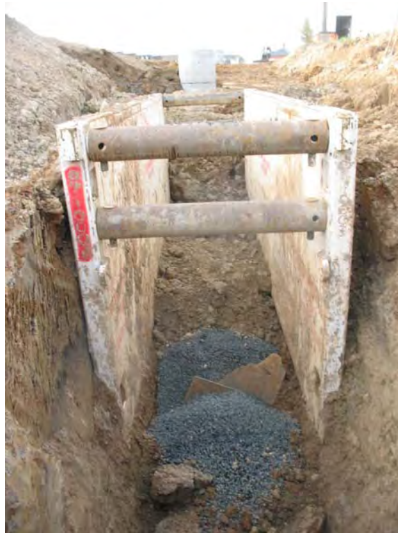
PLATE 26 Trench Box Used in Construction of Sanitary Sewer
