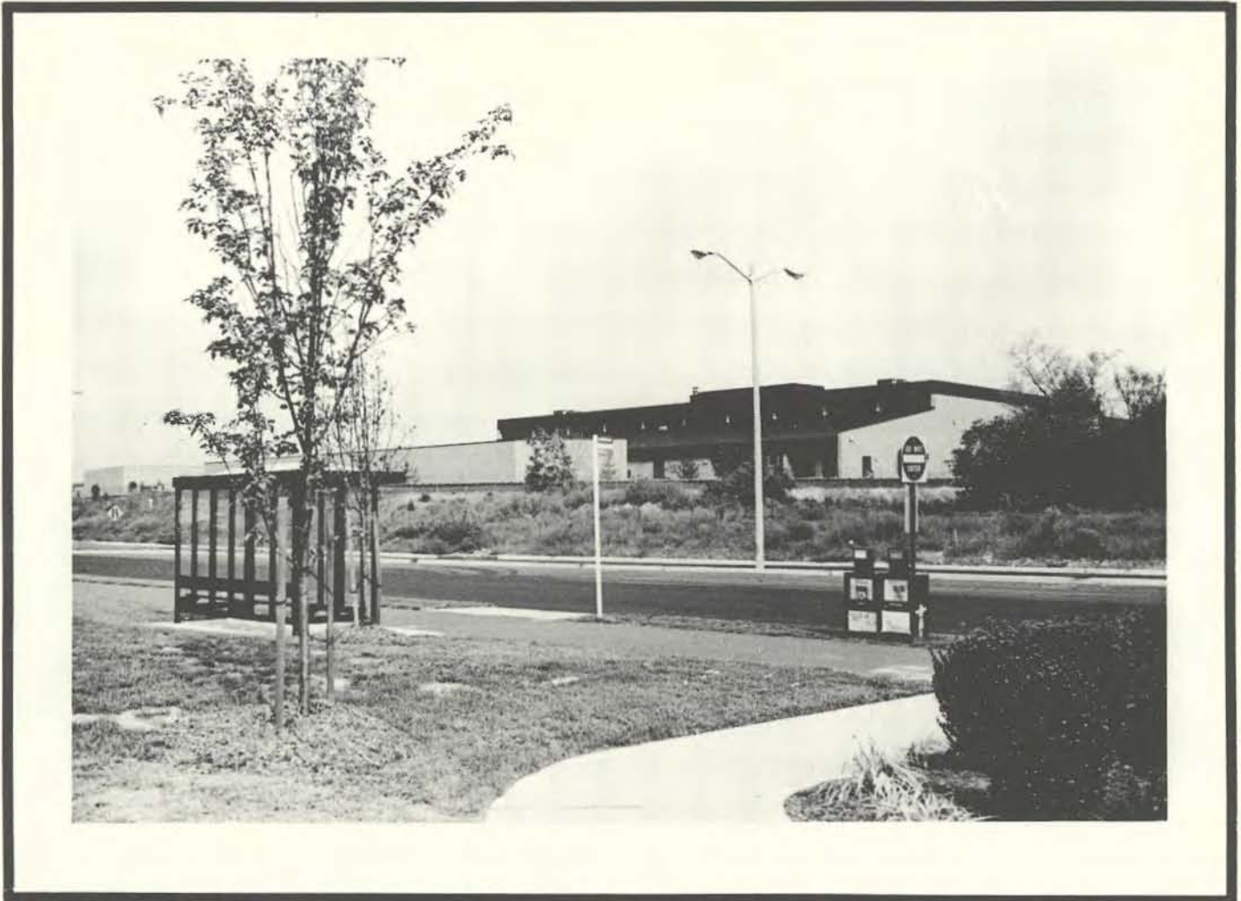
PLATE 10: View North from Eisenhower Avenue toward METRO Inspection Facility.
