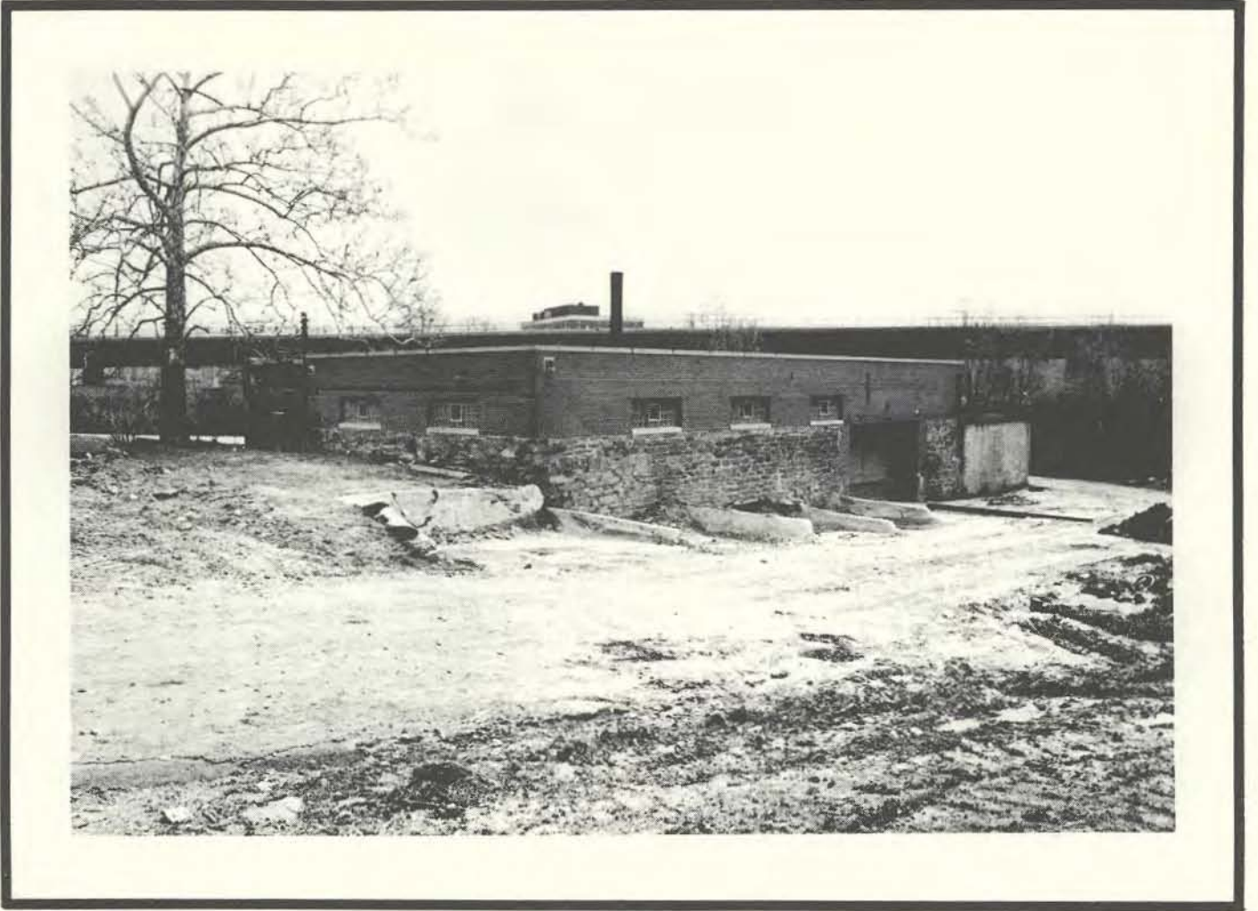
PLATE 3: Alexandria Water Company Building, View to Southeast
