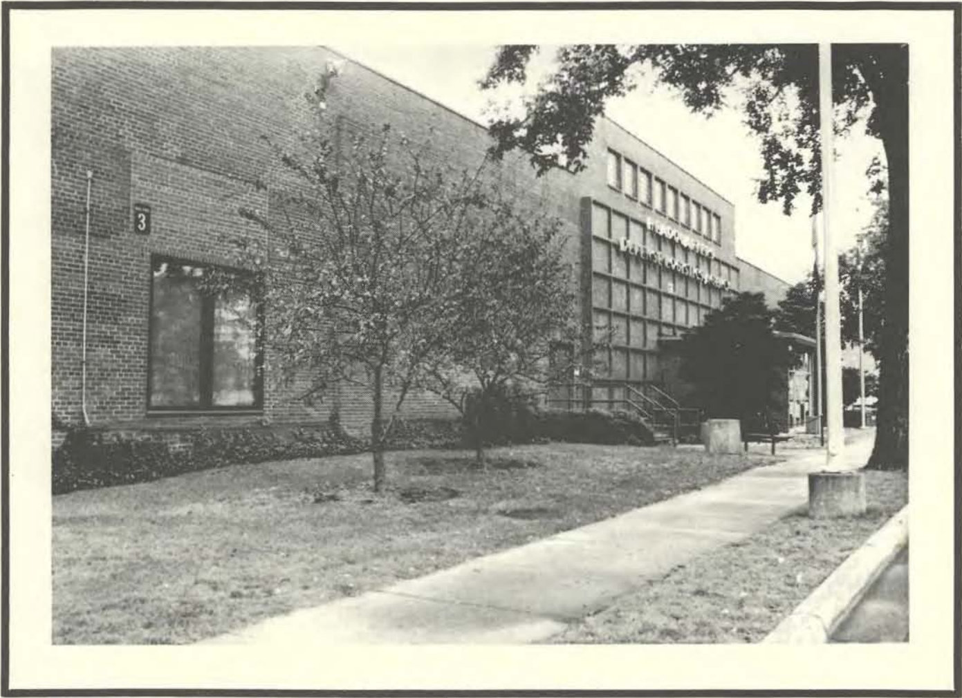
PLATE 19. Cameron Station, Warehouse No. 3, View to Southwest.
