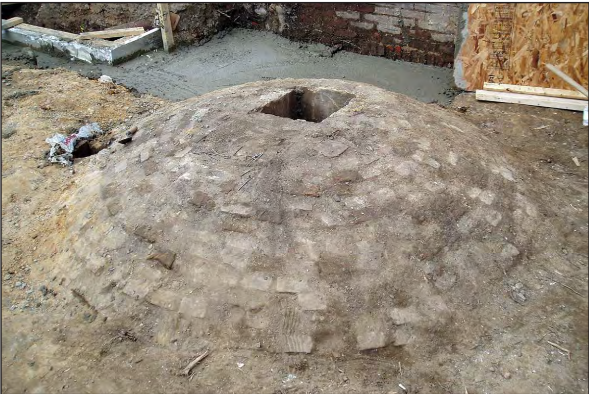
FIGURE 28: Cistern on Cameron Street in Alexandria, with an Intact Brick Dome
