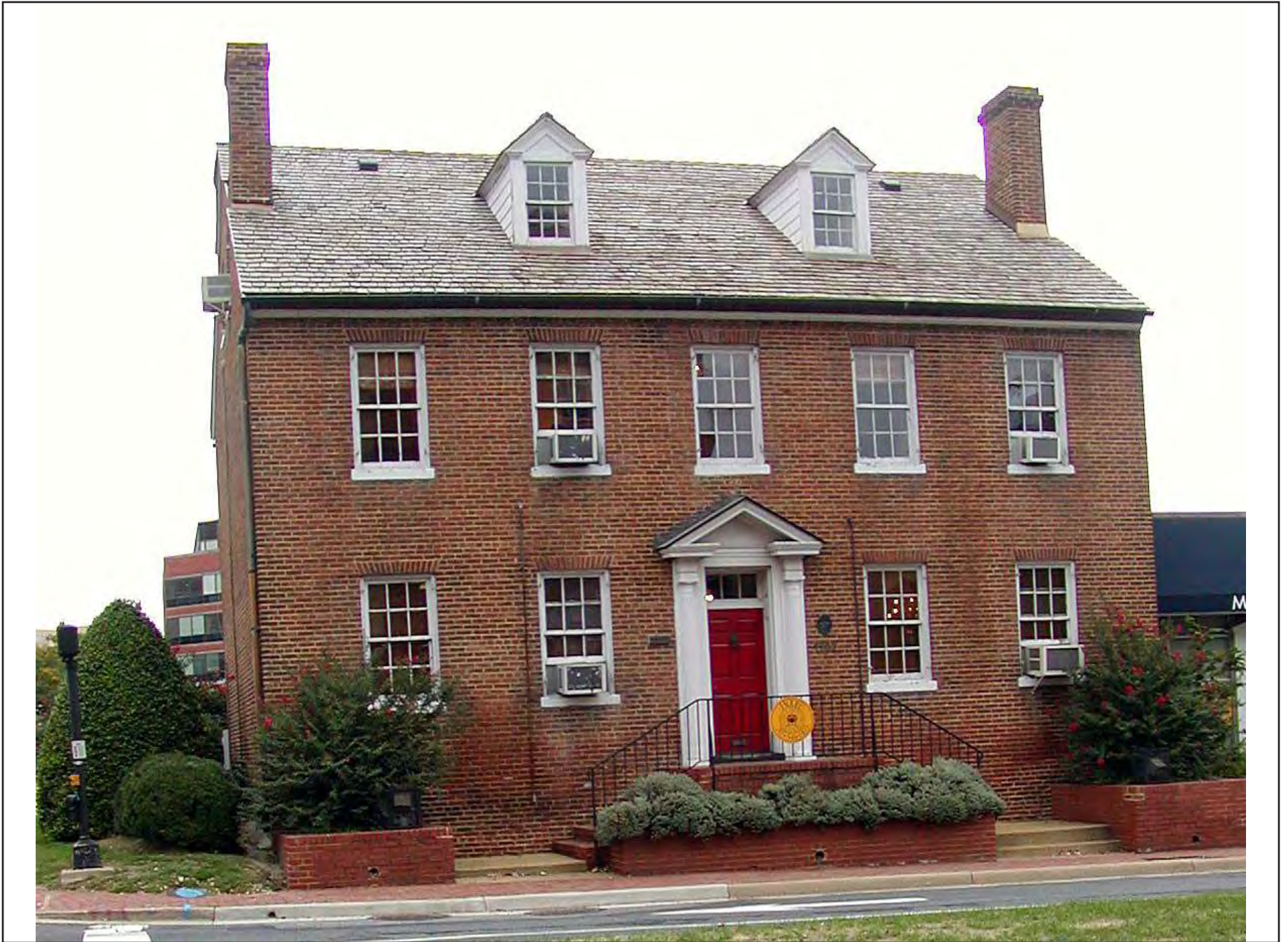
FIGURE 1: Standing Structure at 1707 Duke Street (Bruin's Slave Jail)
