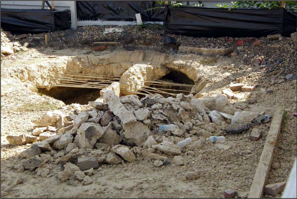
FIGURE 27: Cistern after Removal of Overlying Concrete, September 2008
