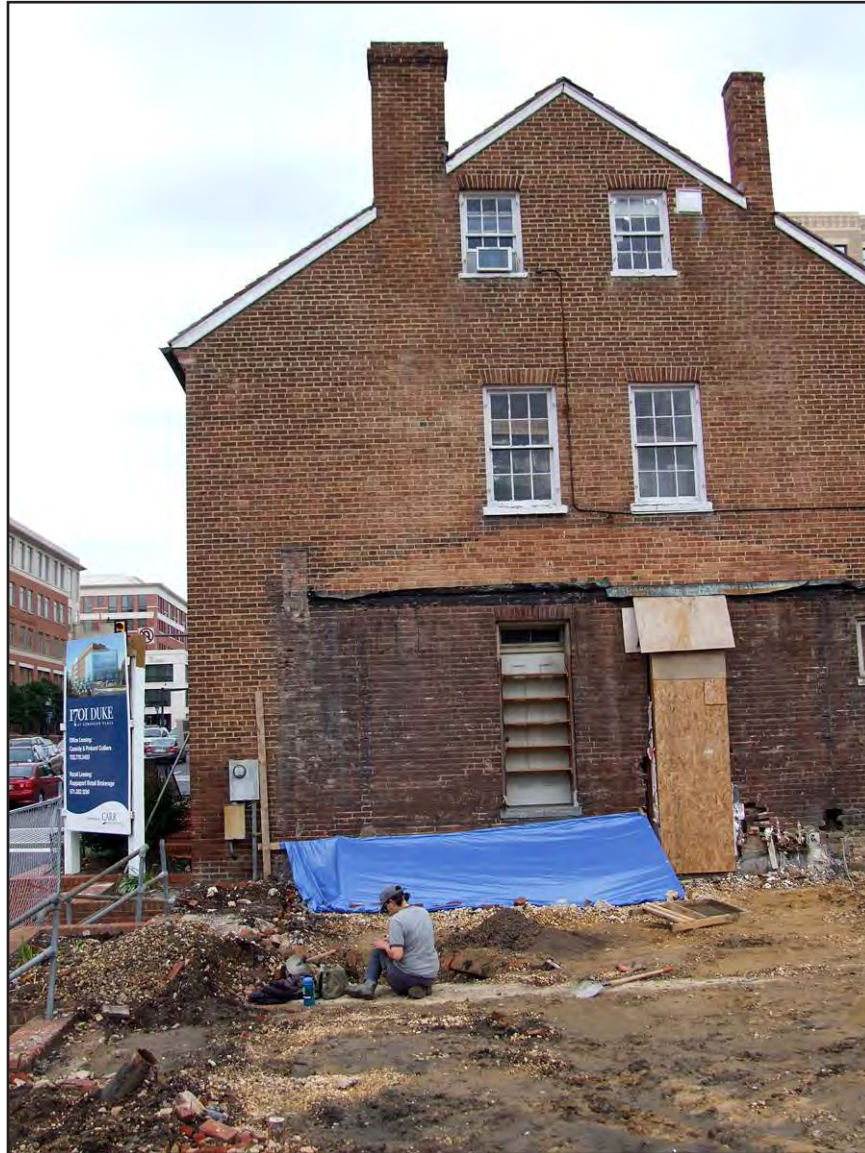
FIGURE 29: South Wall of 1707 Duke Street, with Doors
