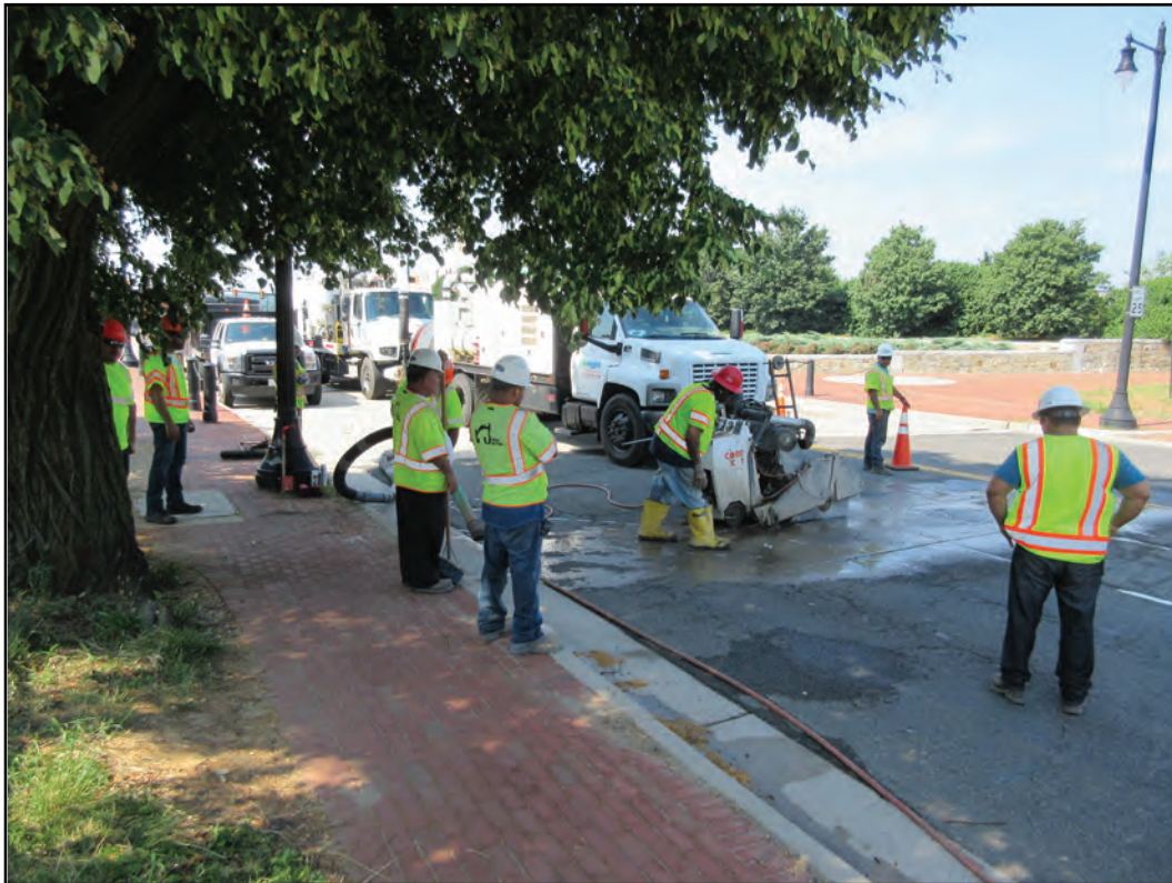
Figure 7-1. View of Pavement Cutting, Facing Southwest
