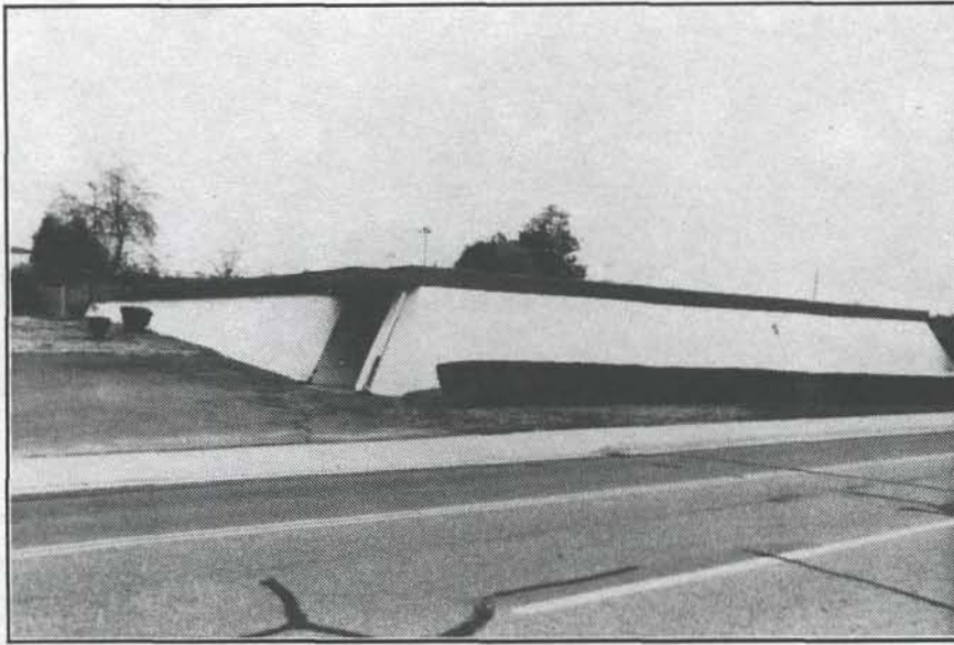
Plate 15. Building 26. View to northeast.
