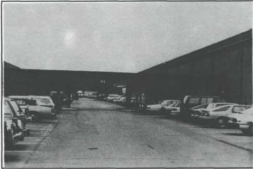
Plate 7. Covered walkways between Buildings 3 and 4. View to south.
