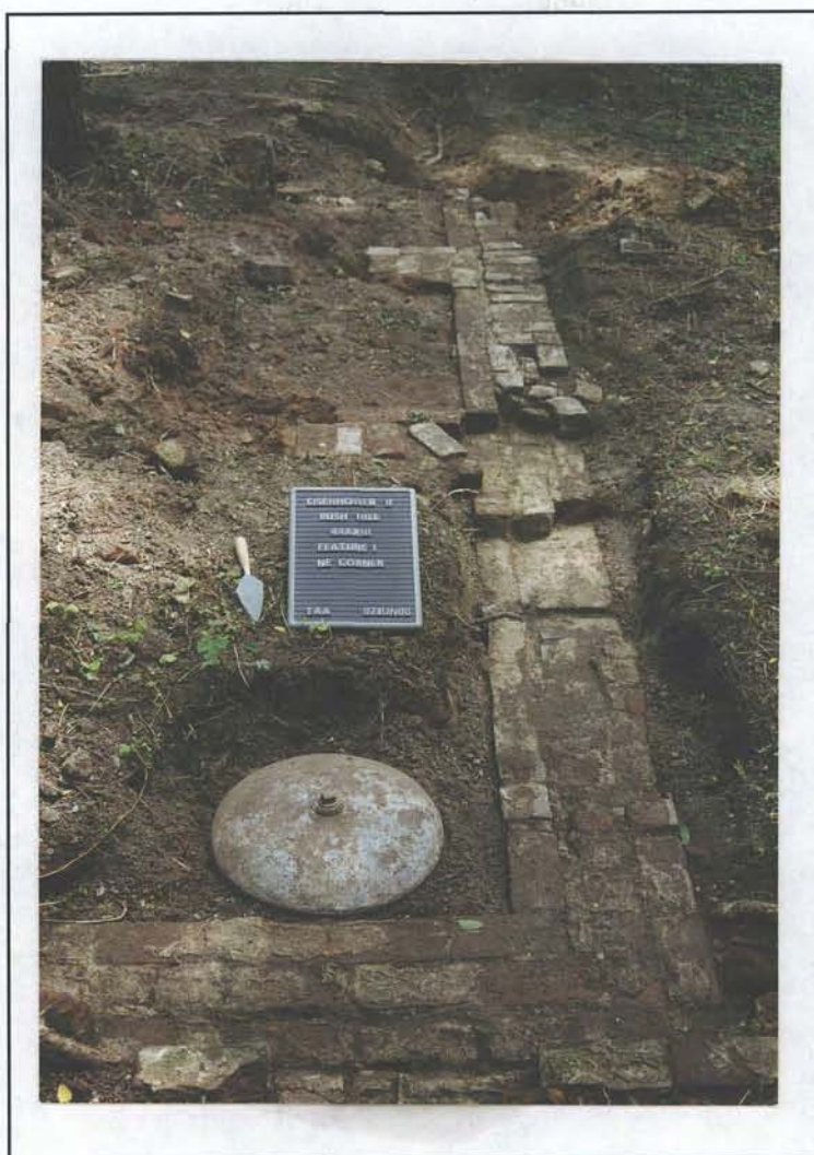
PLATE 7 Feature 1 - Portion of House Foundation (Top of Water Heater Is Visible in Foreground)
