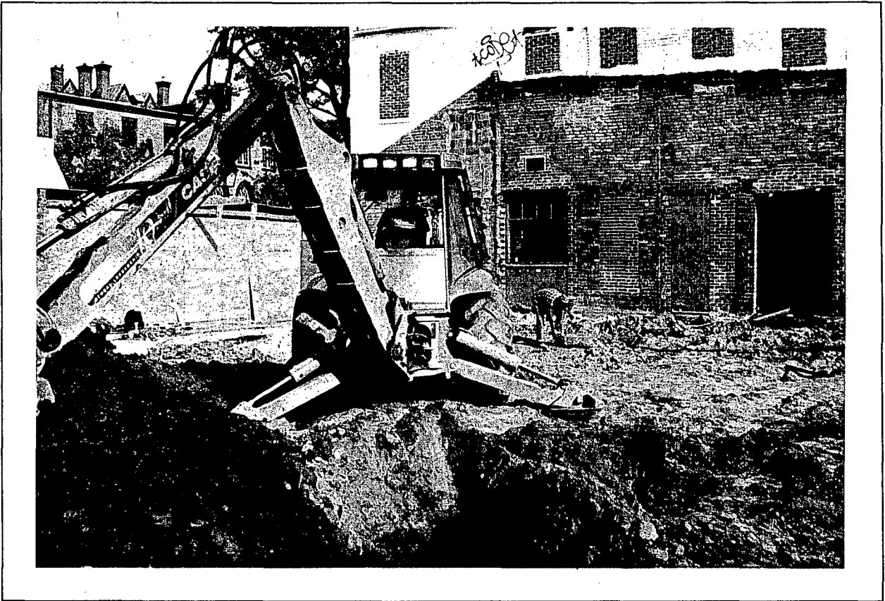
PLATE 1 General View of Excavations
