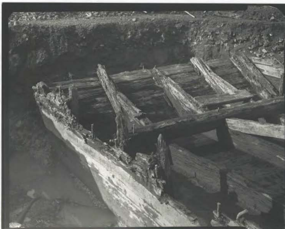
Plate 56. Feature 31, Bow, Ramp Framing
