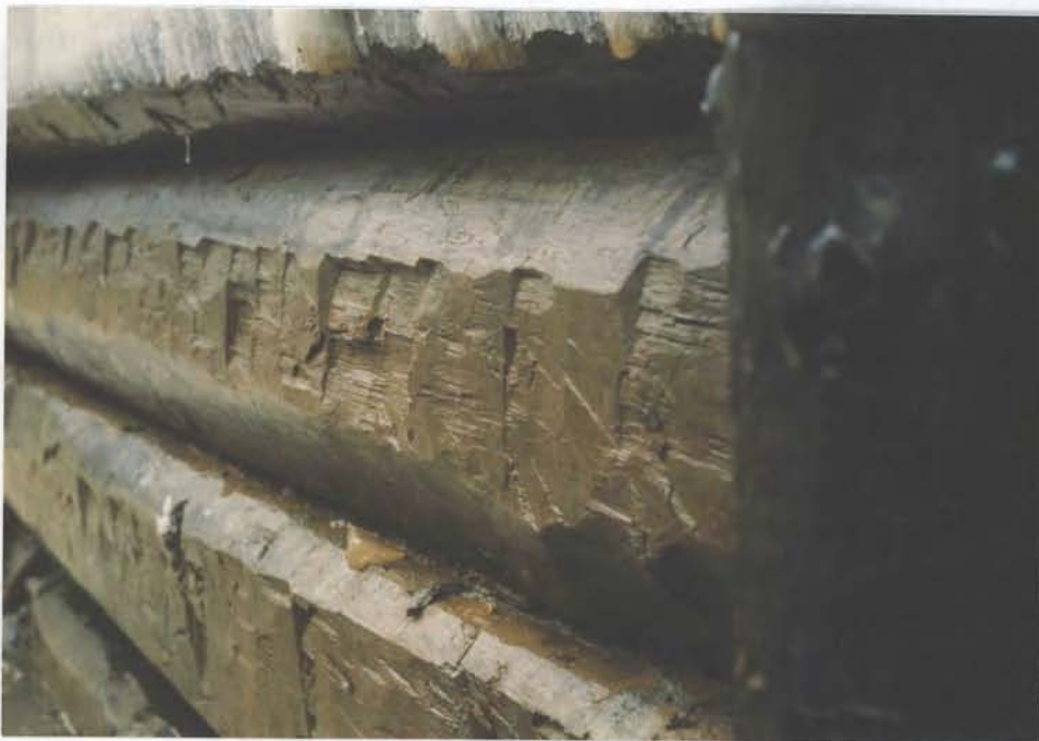
Plate 25. (Below) Detail of Adze-Work, Trench 12G
