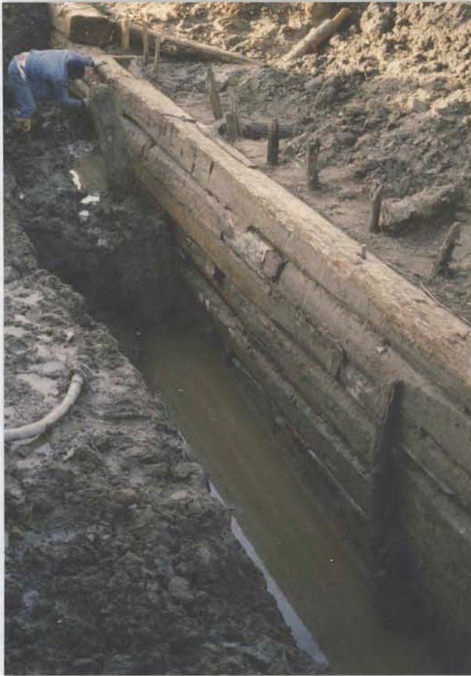
Plate 24. Feature 33--Eighteenth-Century Wharf Bulkhead, Trench 12G
