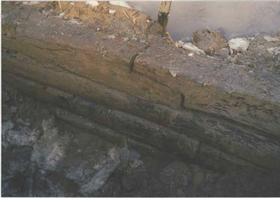
Plate 26. (Above) Detail of Scarf Joint, Trench 12G
