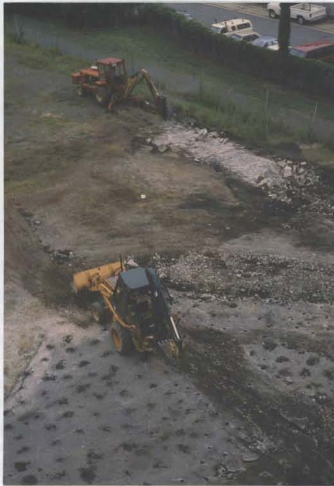
Plate 19. Concrete Slab Removal
