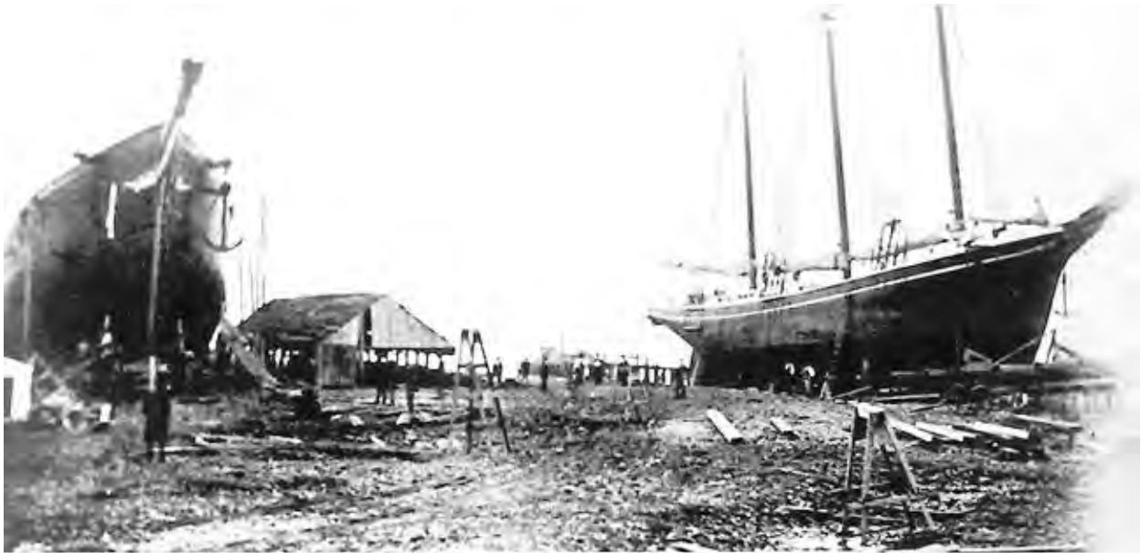
Above: The Alexandria Marine Railway and Shipbuilding Corporation yard, 1880s. Photo courtesy of the Alexandria Library Local History Special Collections. Below: A newspaper advertisement for the Potomac steam packet operated by the Pioneer Steamboat Company of which Robert Portner was co-owner and president.
