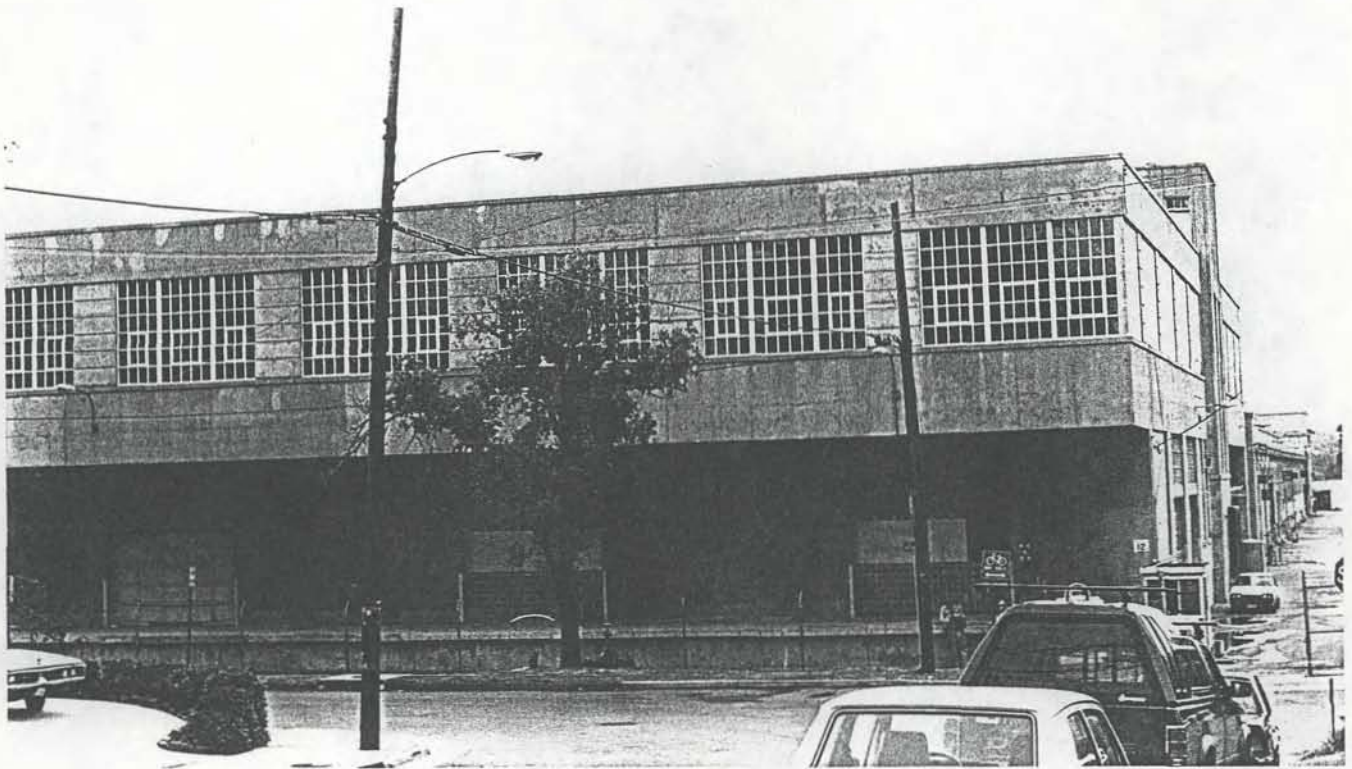
Photograph of a portion of the west elevation (South Union Street view) of Building #12, showing loading dock.
