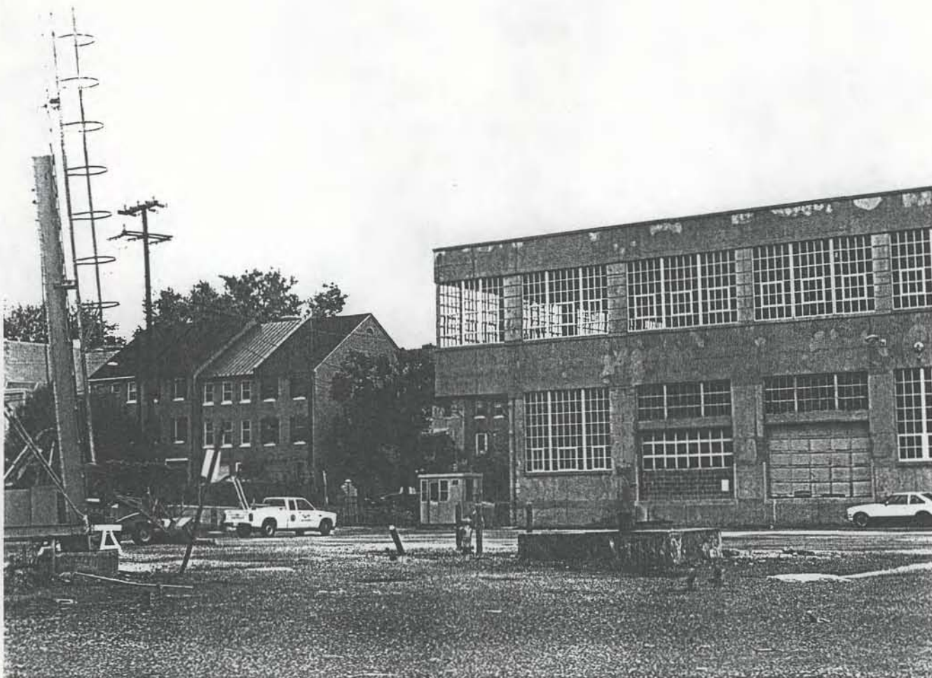
Photograph of the southwest corner of Building #12, with a portion of the water tower supports in the foreground.
