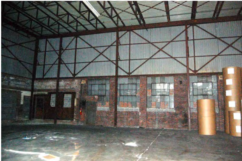
Figures 41 & 42. Interior of RTWC warehouse at corner of South Union and Duke Streets. When RTWC acquired the former Southern Iron Works property, it used the 1938 fabricating building with its two-story section along South Union Street (remains on left) and barrel-vaulted, one-story building (ghost marks from the barrel-shaped roof are seen on the brick structure, and the Duke Street elevation is seen on right). In 1962, the RTWC spanned these under one roof. (History Matters, LLC; April 2014)
