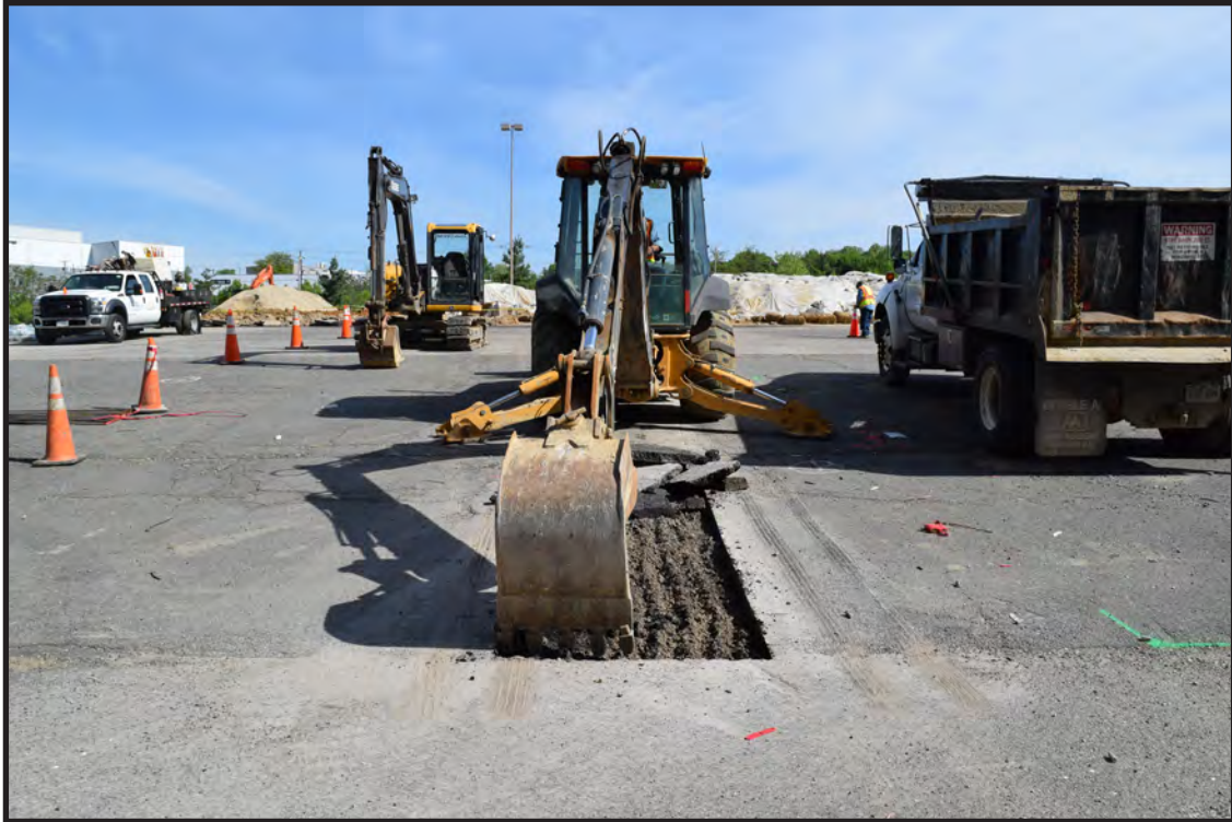
Figure 2.9 Photograph showing backhoe removing the asphalt surface at Trench 2, view north
