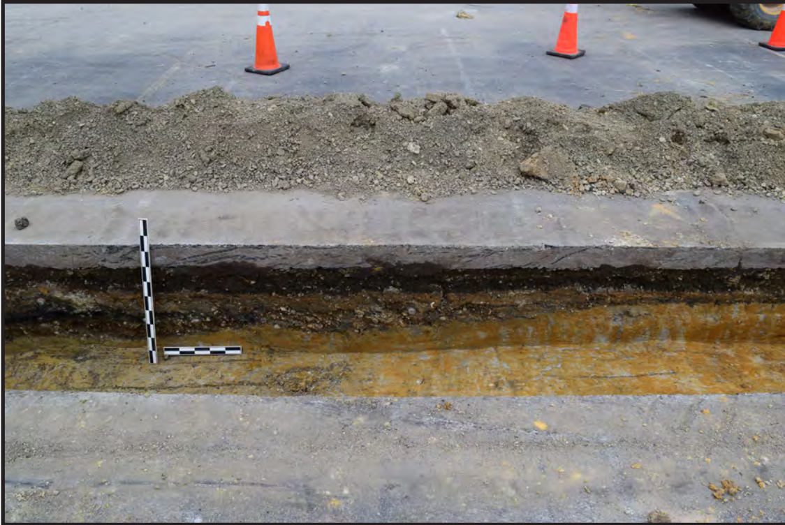
Figure 3.15 Trench 4: Photograph showing Section 10-15 m, profile west (78 cm below surface)
