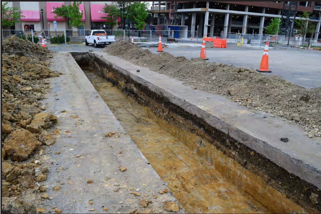
Figure 3.16 Trench 4: Photograph showing oblique view of trench, profile west
