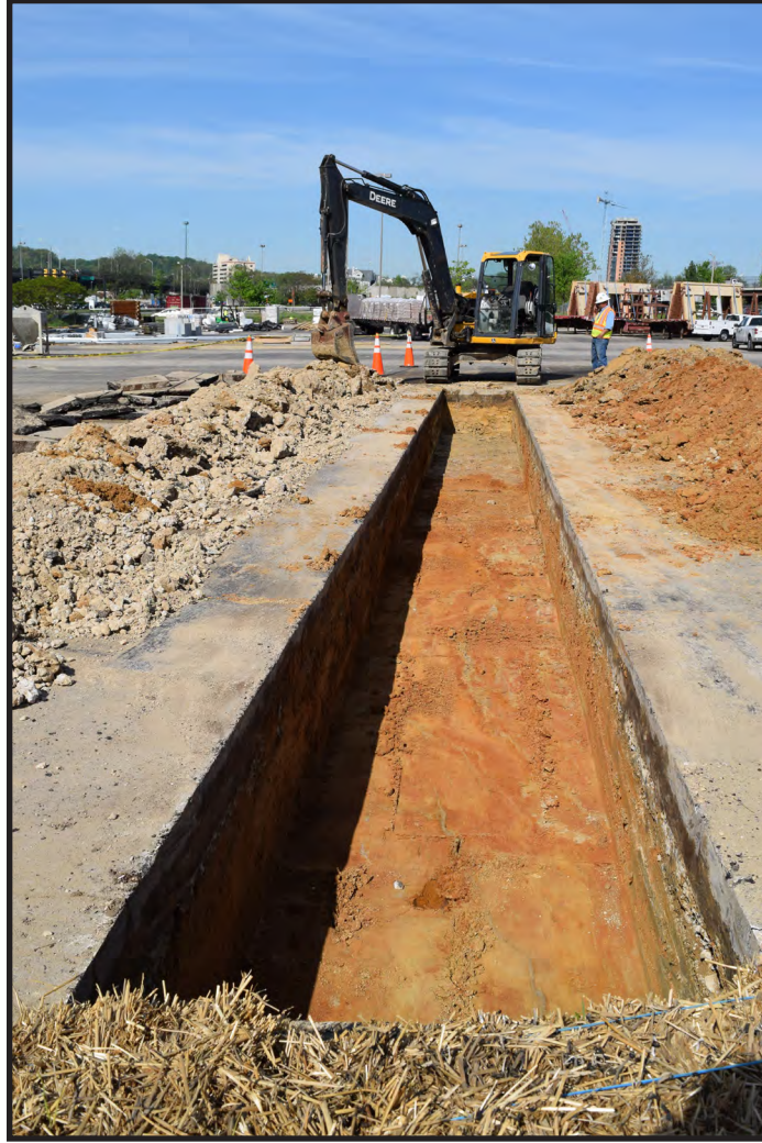
Figure 3.21 Trench 5: Photograph showing subsoil, plan view facing west (78 cm below surface)
