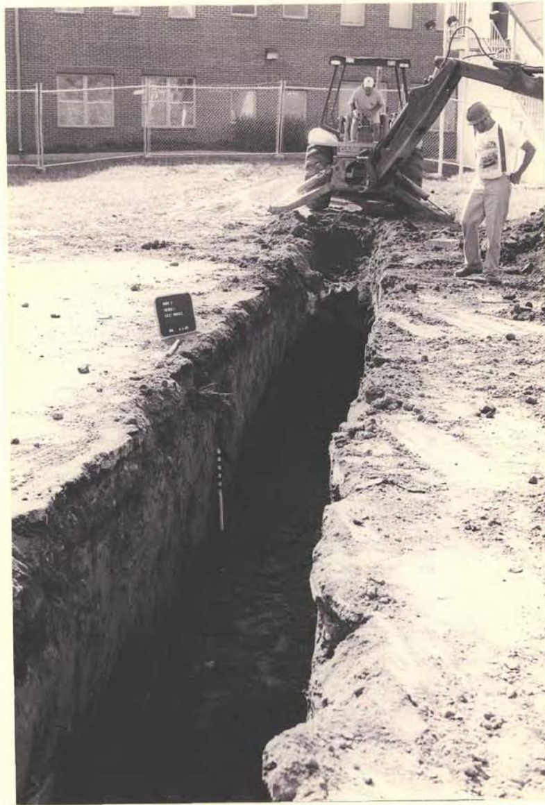
Figure 6. Overview of excavation of trench 1, facing east.
