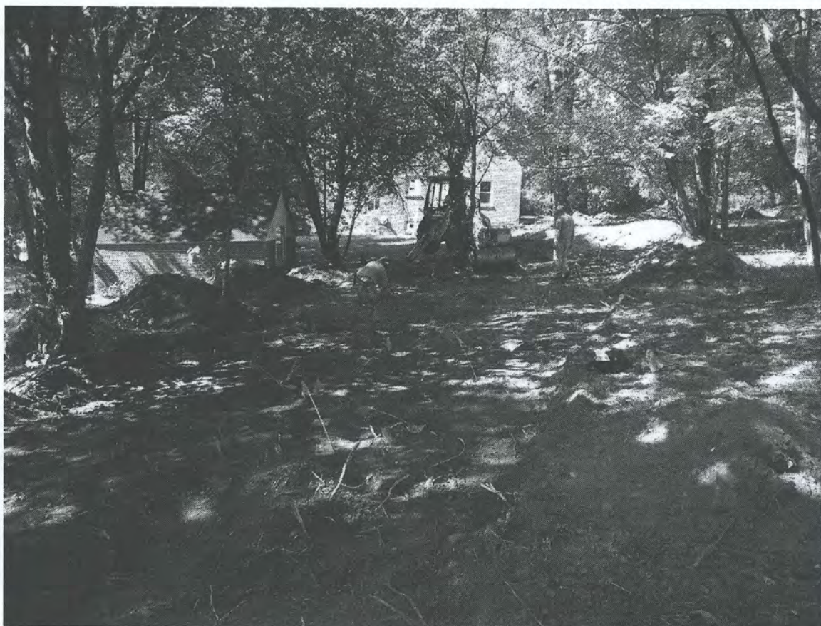
Figure 6. Mechanical stripping and metal detection, facing west.
