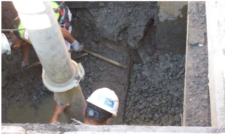
Figure 21: The Strand Utility Trench
