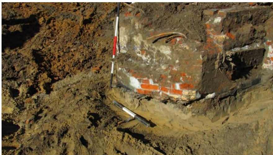
Figure 17: Site Leveling #2, 20 th Century Brick and Mortar Footers
