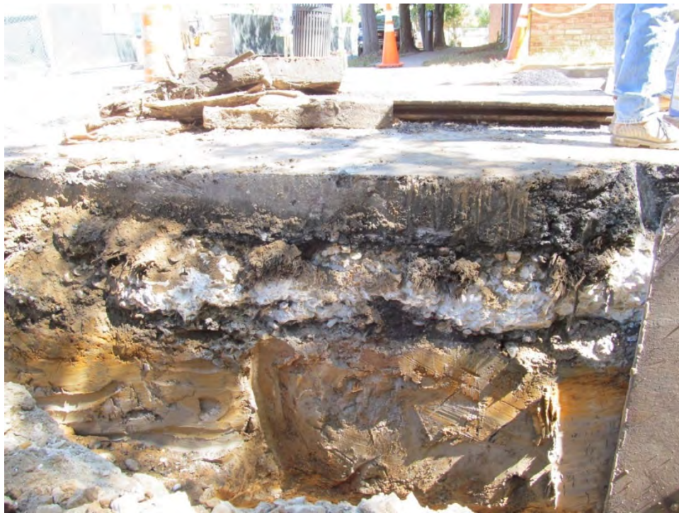
Figure 18: Union Street Utility Trenching
