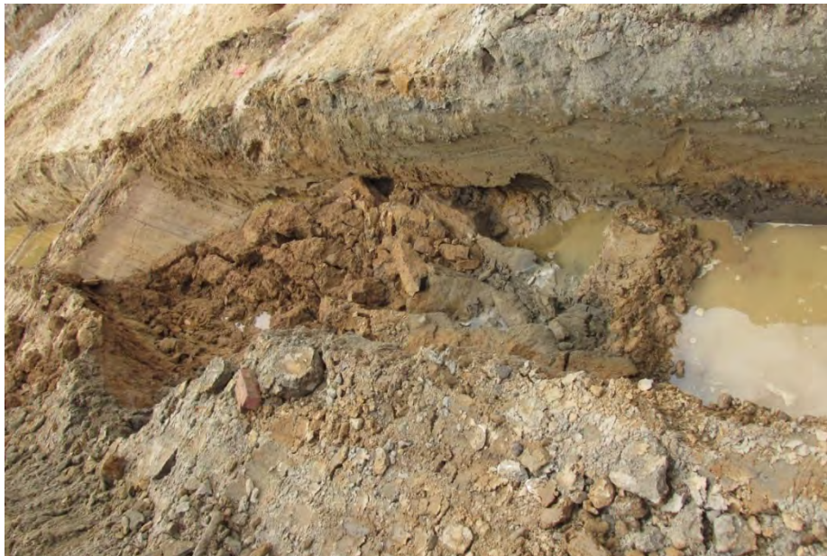
Figure 13: Trench 2, Part 2, Collapsed Wall
