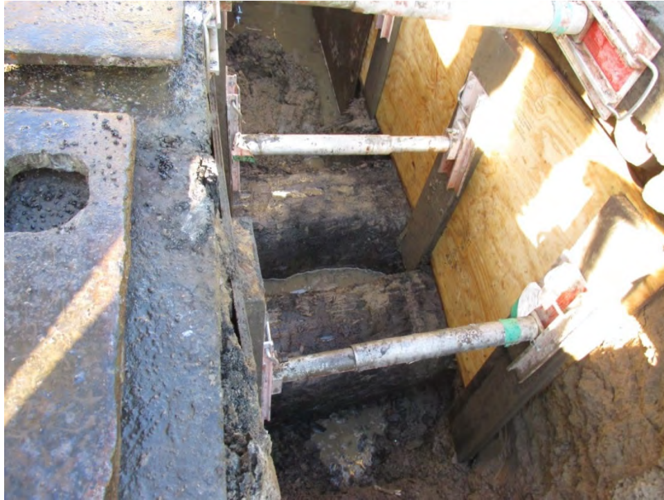
Figure 19: Duke Street Utility Trenching
