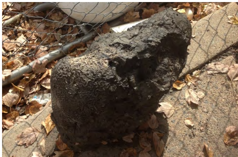
Figure 22: The Strand Utility Trench, One Wooden Log Removed
