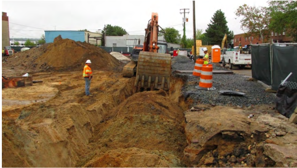
Figure 10: Piling Trench Monitoring
