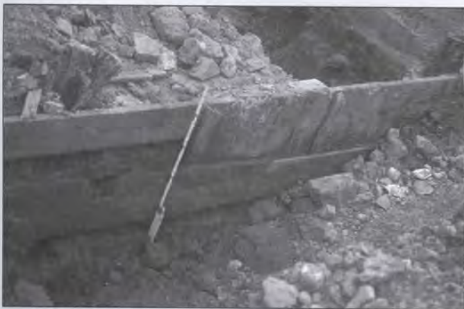
Remains of wooden coal storage shed
