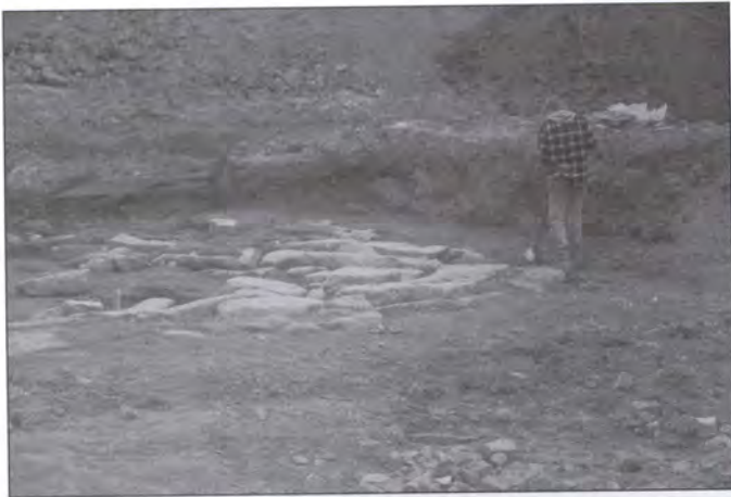
Wharf surface covered with large, flat stones
