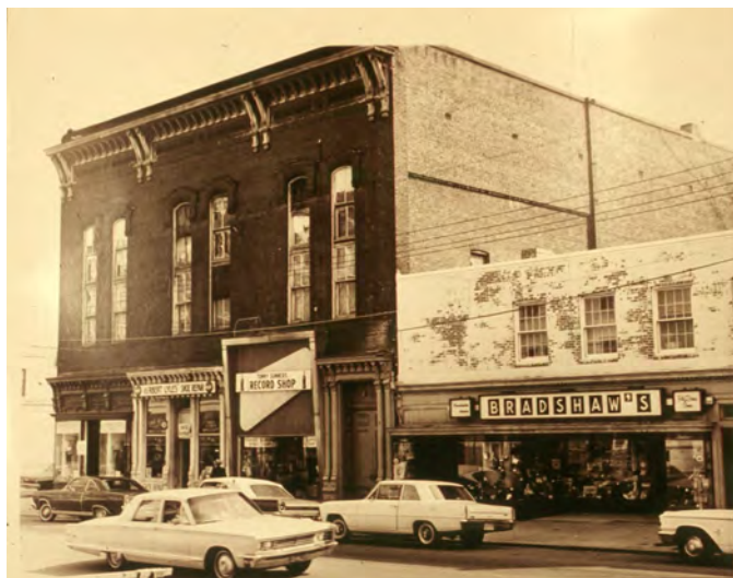
Figure 28 - King St frontage of Lannon's brick building , 1967 (ALEXANDRIA ARCHAEOLOGY COLLECTION)
