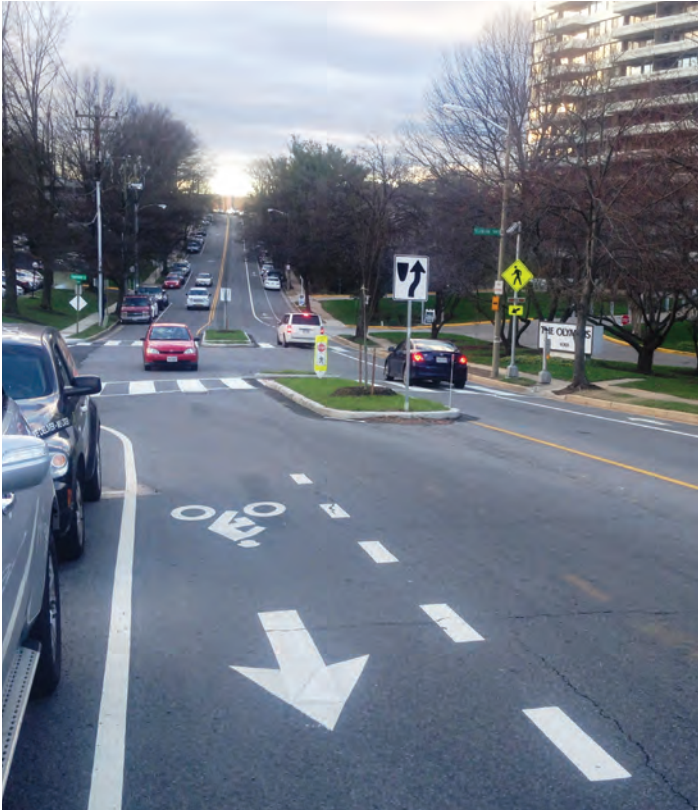
Example of an Existing Complete Street in Alexandria (Stevenson Ave)
