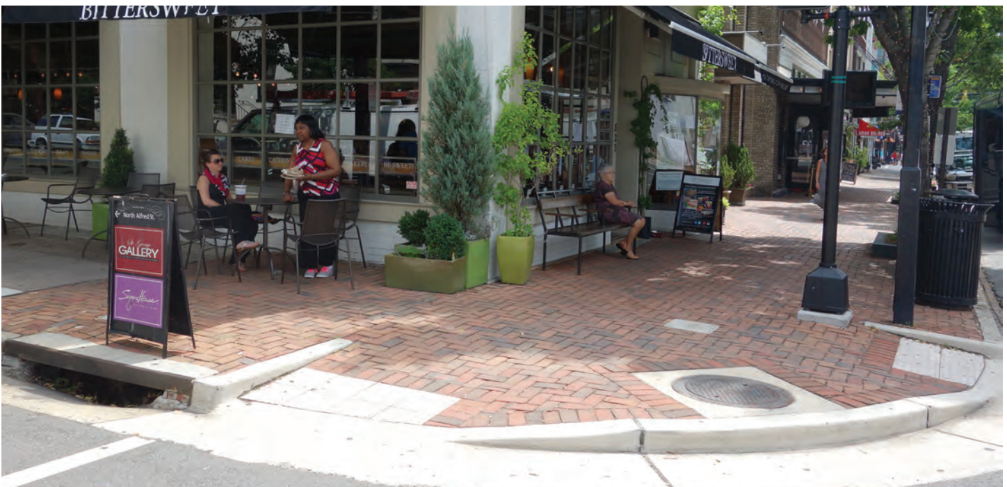
Recently Installed Sidewalks and Existing Curb Ramps in Alexandria
