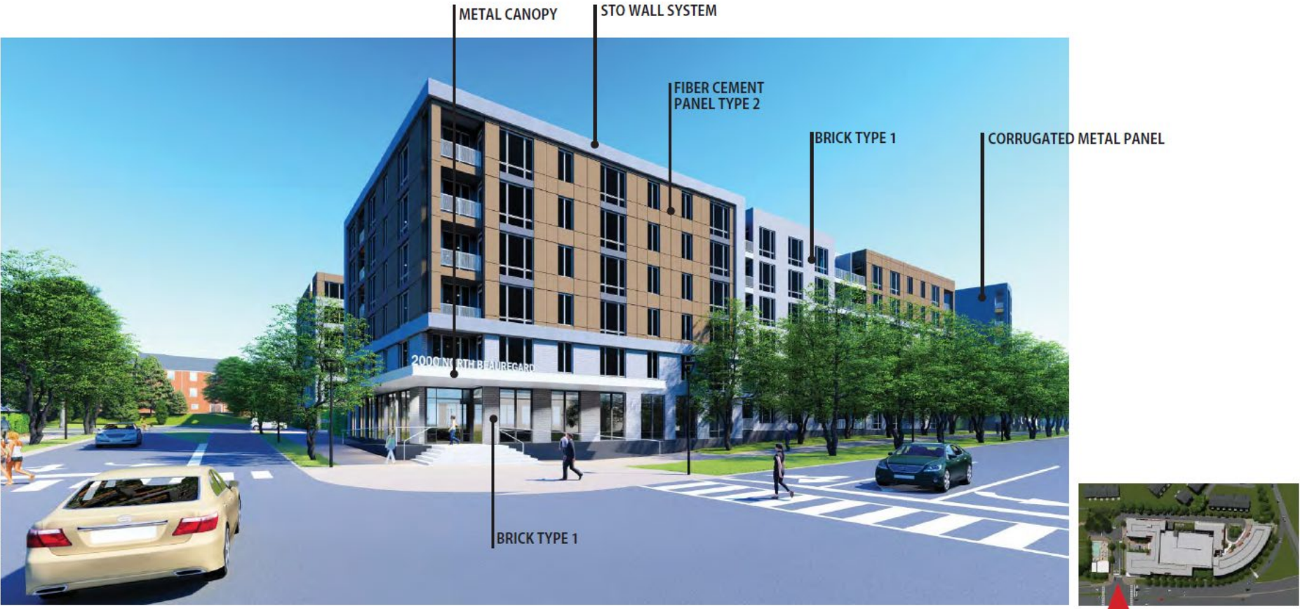
Figure 4: West building wing and primary building lobby at the intersection of Mark Center Drive and N. Beauregard Street, as seen from N. Beauregard Street.
