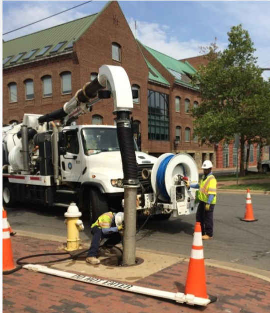
Catch basin cleaning, Prince Street
