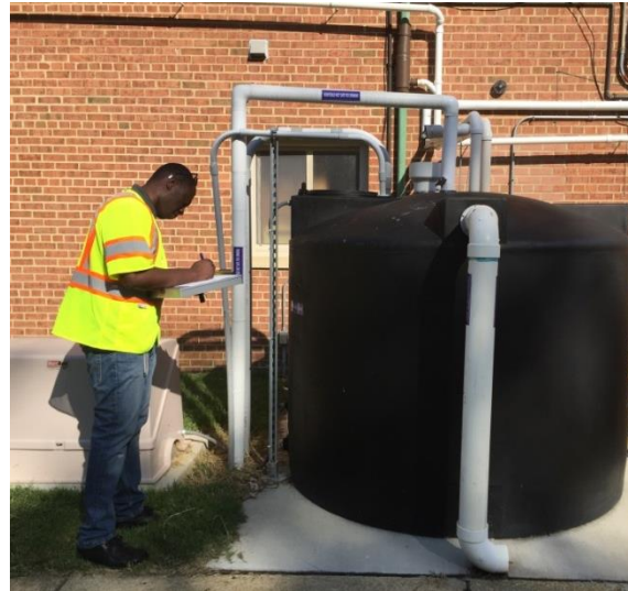
BMP Inspection, Fire Station 206
