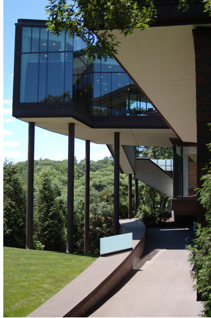
COLUMN AT CANTILEVERED CORNER
