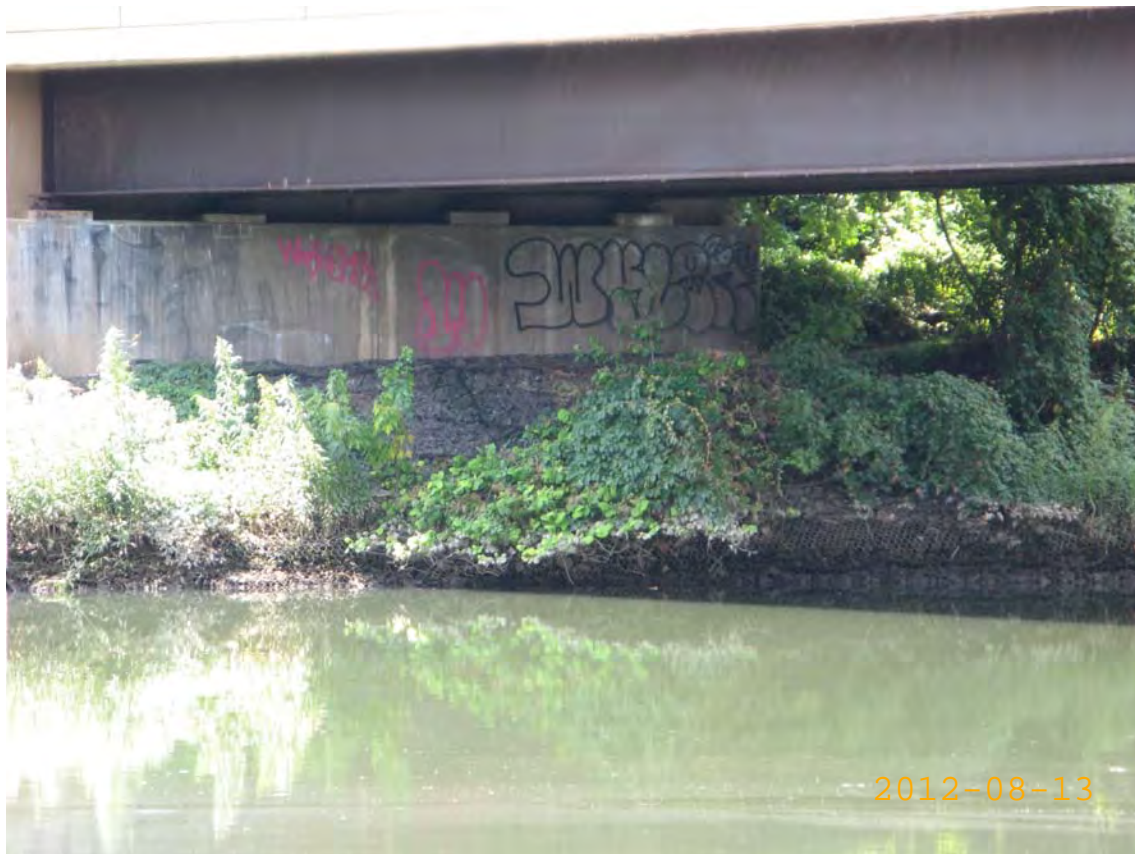
Photograph 5. Area 2 - View of Area 2 southern bank of Four Mile Run on August 13, 2012, during habitat survey. Note gabion baskets that line stream banks from mean low water to above mean high tide.
