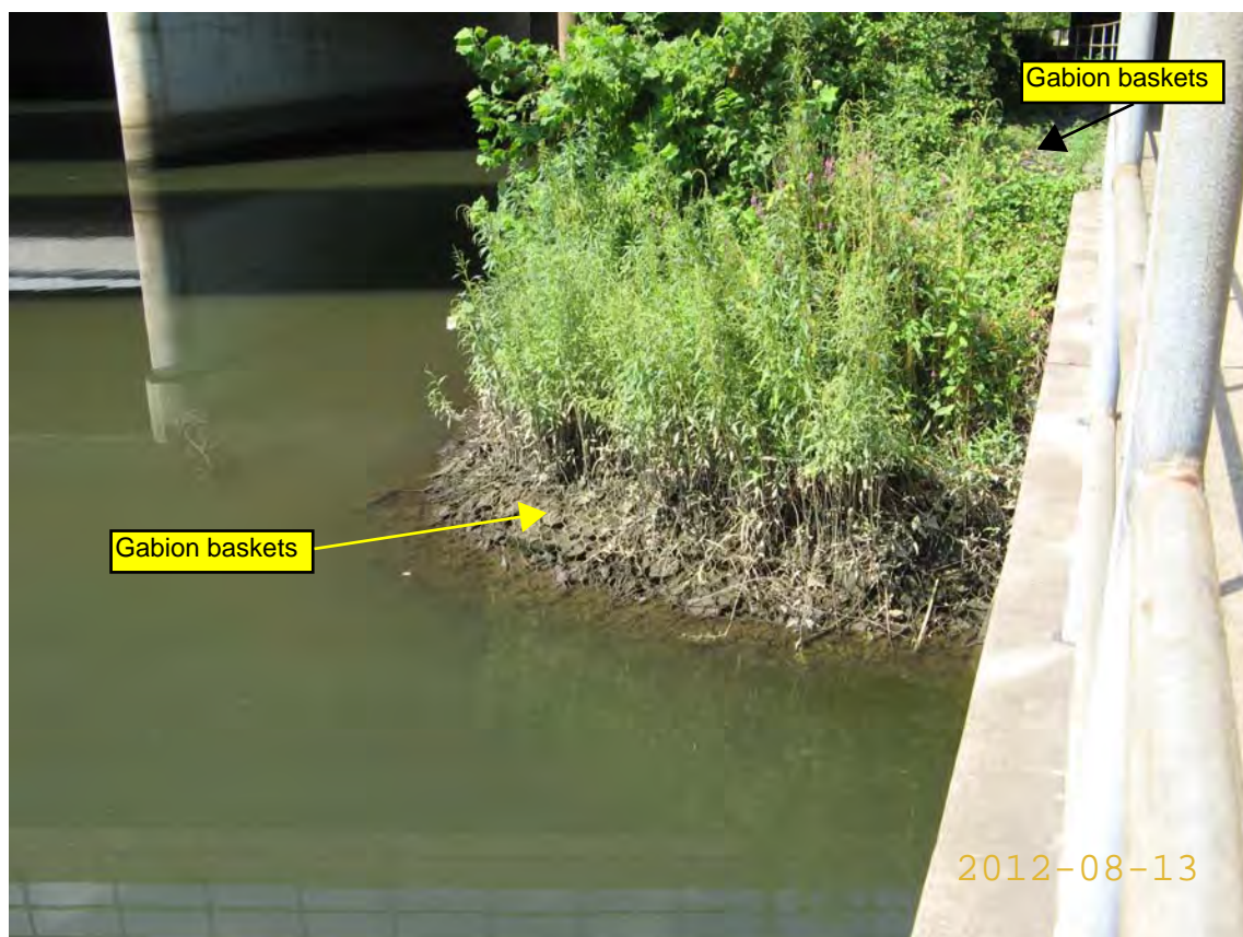
Photograph 4. Area 1 - View of Area 1 and Area 2 west side connection on August 13, 2012. Note gabion baskets at extending from below the water and extending above mean high tide.
