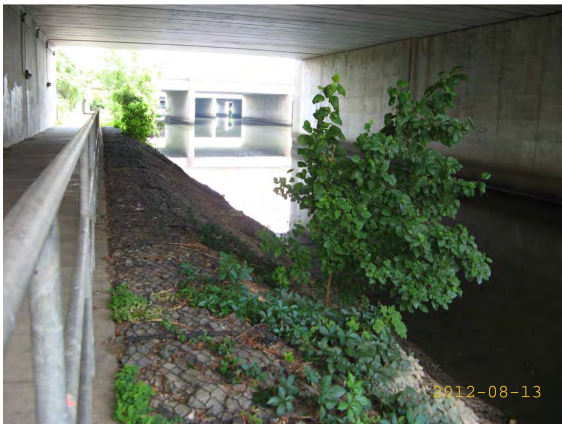
Photograph 6. Area 2 - View of Area 2 northern bank of Four Mile Run on August 13, 2012, during habitat survey. Note gabion baskets that line stream banks from mean low water to above mean high tide..
