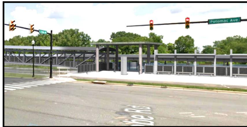
Glebe Road Entrance
