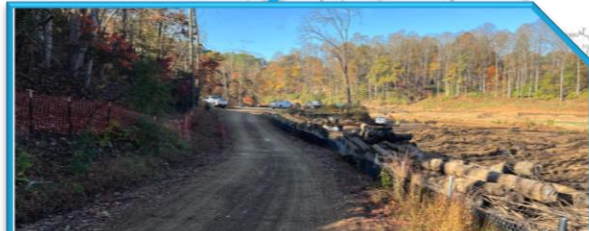
Construction Access/Timber Matting
