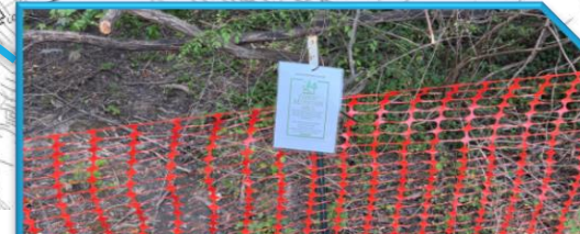
High Visibility/Tree Protection Fence
