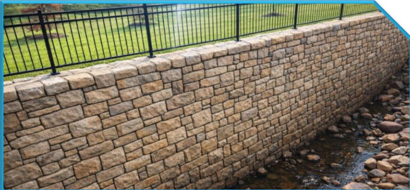
Gravity Wall with Safety Railing
