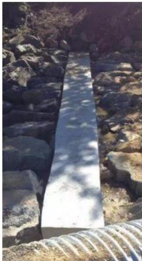
Sanitary sewer in concrete encasement protected by boulders
