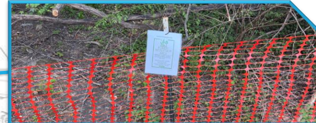
High Visibility/Tree Protection Fence
