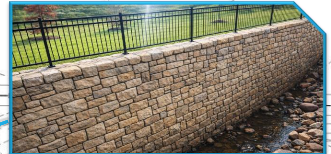
Gravity Wall with Safety Railing
