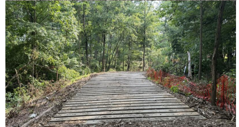
Deck Mat/Construction Access Road
