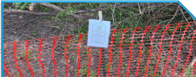
High Visibility/Tree Protection Fence
