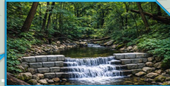
Boulder Weir and Pool
