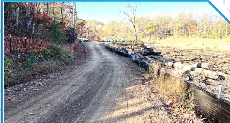
Construction Access/Timber Matting
