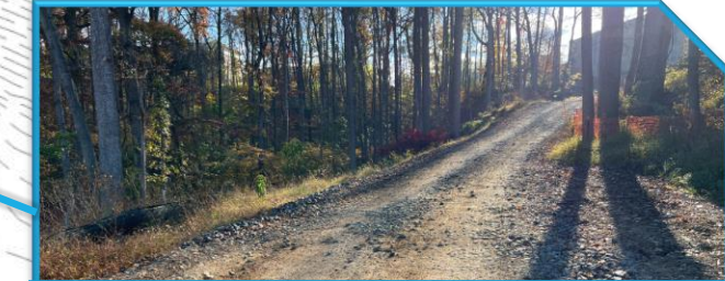
Construction Access/Timber Matting
