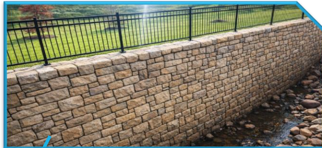
Gravity Wall with Safety Railing
