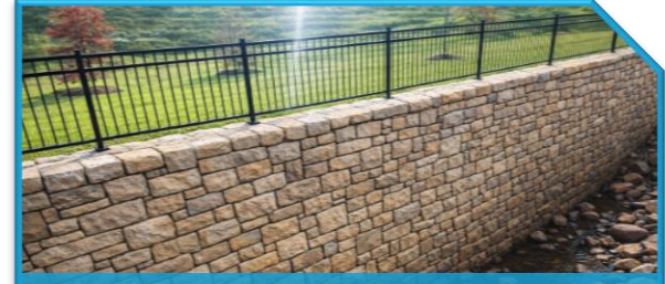
Gravity Wall with Safety Railing
