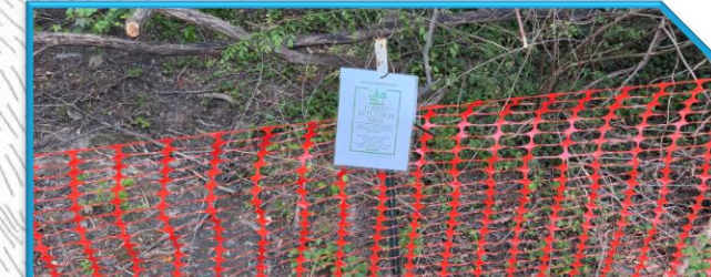
High Visibility/Tree Protection Fence
