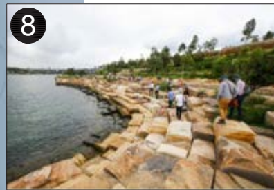
BLOCK SEATING AND SHORELINE STABILIZATION
