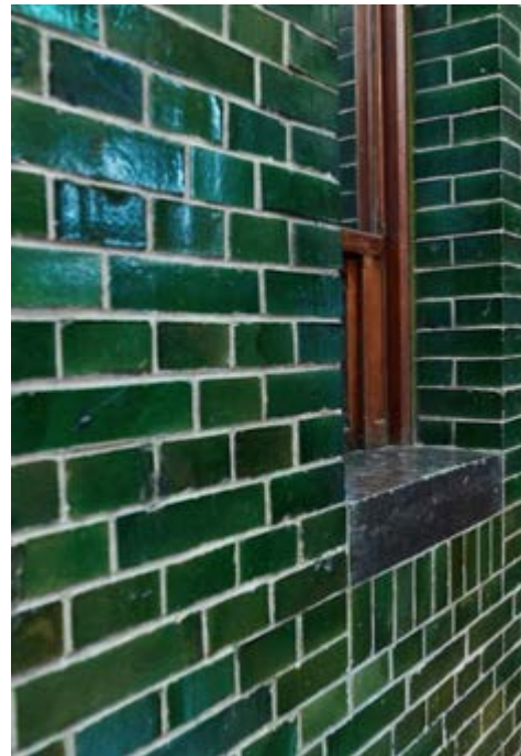
GLAZED BRICK/TILE LOGGIA
