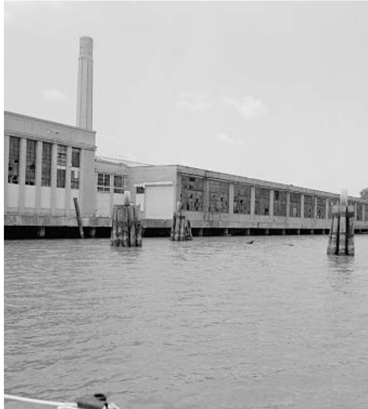
Demolished Ford Plant/ Waterfront Industrial History
