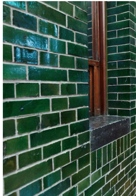
GLAZED BRICK/TILE LOGGIA
