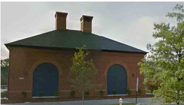
Images depict types of potential pump station facility designs. Left: existing facility located in South Potomac Yard. Right: integrated facility concept.
