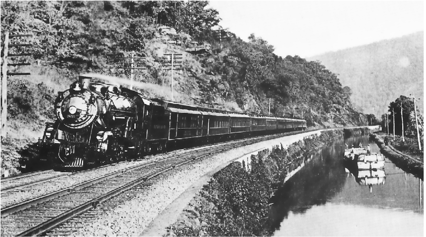
Image of railroad corridor along the Alexandria Canal
