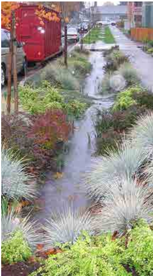
Above: Stormwater management facility.
