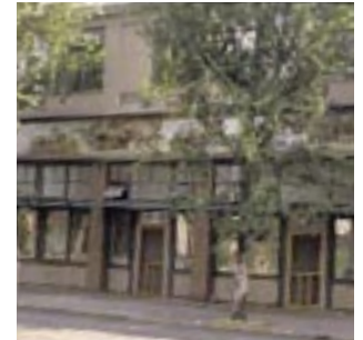
Example of Artists’ Loft Building, Artspace Projects Inc.
