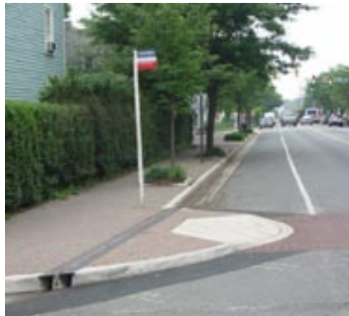
Example of Existing Bulb-out
