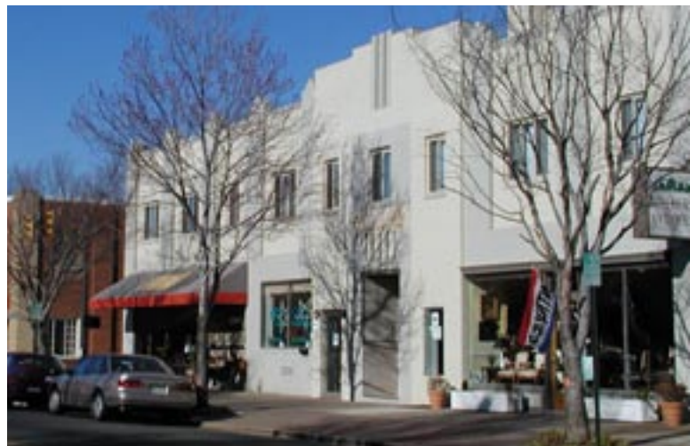
Figure 6.16 Architectural detail and interest
