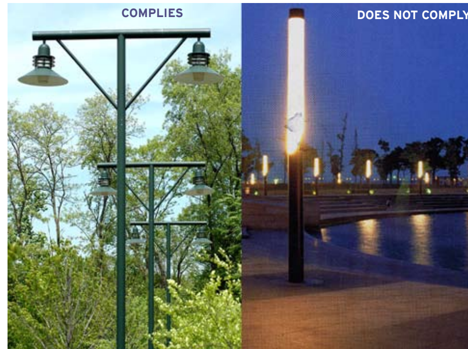
TWO EXAMPLES OF LIGHTING: ONE COMPLIES WITH “DARK SKIES” STANDARDS, THE OTHER DOES NOT COMPLY
