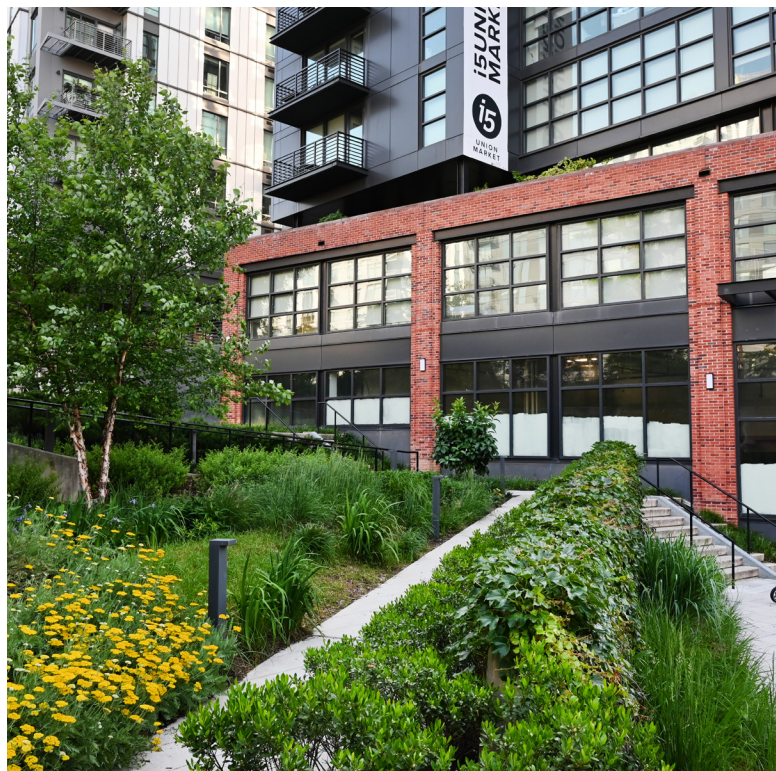
The topography can be embraced and integrated into redevelopment.
