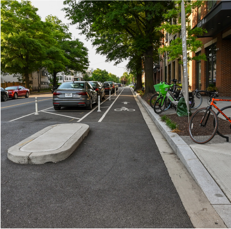
Bike lanes will ensure residents can safely navigate the neighborhood by bicycle.
