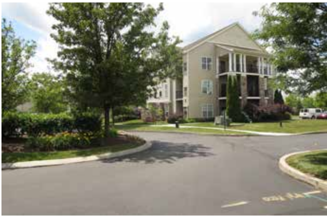
A traffic circle with attractive landscaping calms traffic through the multifamily residential portion of The Point at Pennbrook Station development.
