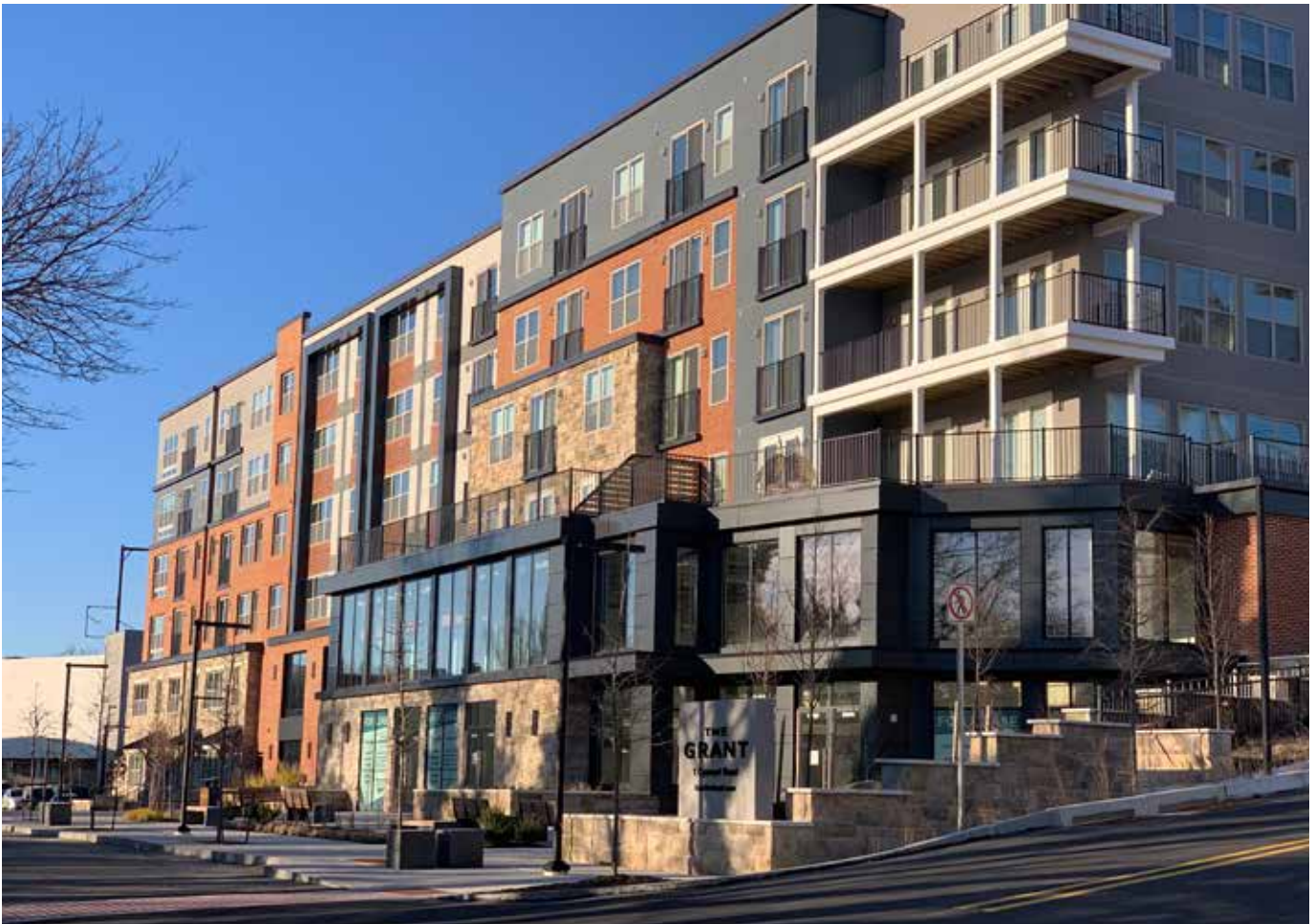
The Grant development near the Bala train station in Lower Merion Township incorporates a prominent retail space on the corner. A pedestrian plaza provides landscaping and seating areas adjacent to the retail space.
