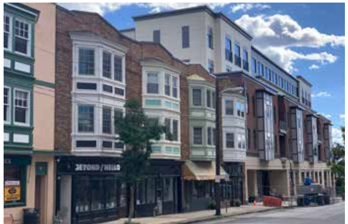
The Cricket Flats development in Ardmore utilizes a building stepback along the main building frontage above the third story to create a context-sensitive transition between the new construction and the existing three-story buildings on the block.
