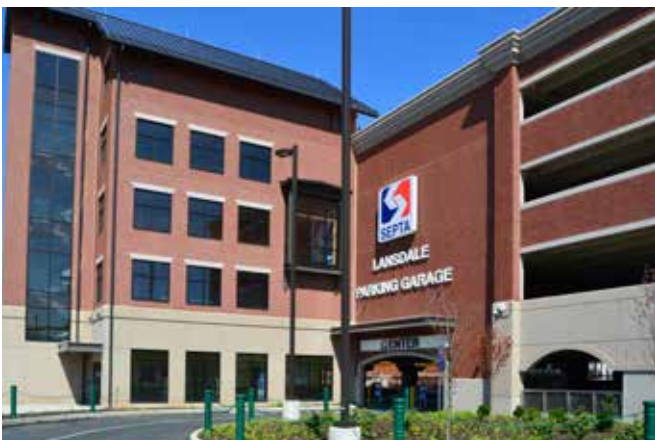
The parking garage at the Lansdale Station opened in 2017. A pedestrian bridge connects the garage to the Madison Lansdale Station mixed-use development across the railroad tracks.
