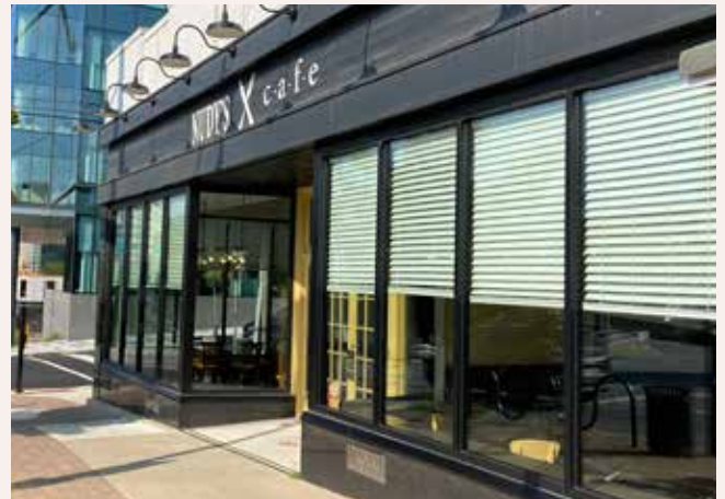
Fayette Street, Conshohocken Borough
