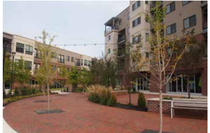
Although the Madison at Lansdale Station development is primarily residential, the building closest to the train station is mixed-use, with ground floor commercial space that fronts onto public gathering space, with apartments above.
