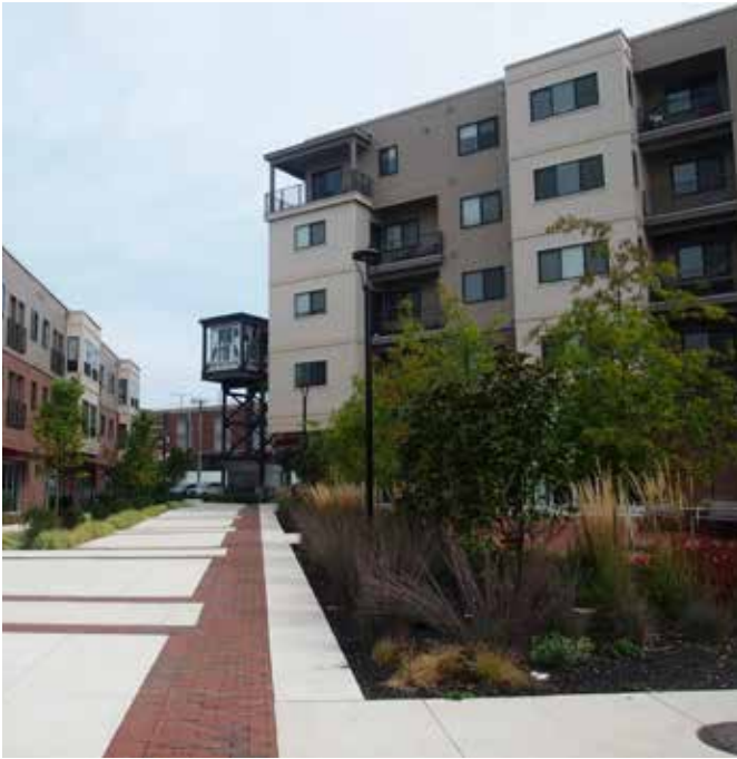
A linear plaza connects Madison Street and the pedestrian bridge to the Lansdale SEPTA parking garage to the north.
