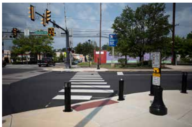
Continental-style crosswalks and pedestrian push-button signals improve pedestrian access between The Station at Willow Grove development and the Willow Grove train station.
