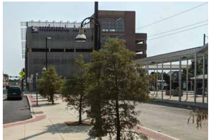
A parking garage accommodating 513 vehicles opened at the Norristown Transportation Center in 2008. The garage services riders on Regional Rail, the NHSL, and eight SEPTA bus routes.
