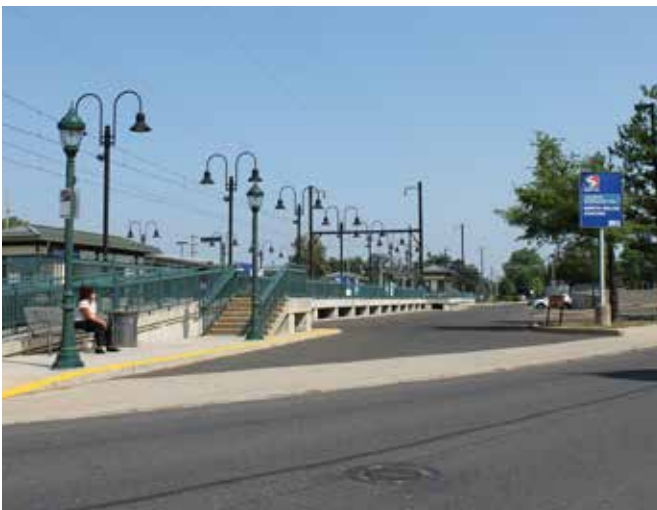
The land closest to the North Wales Station in North Wales Borough is currently used for commuter parking, as is common across Montgomery County.
