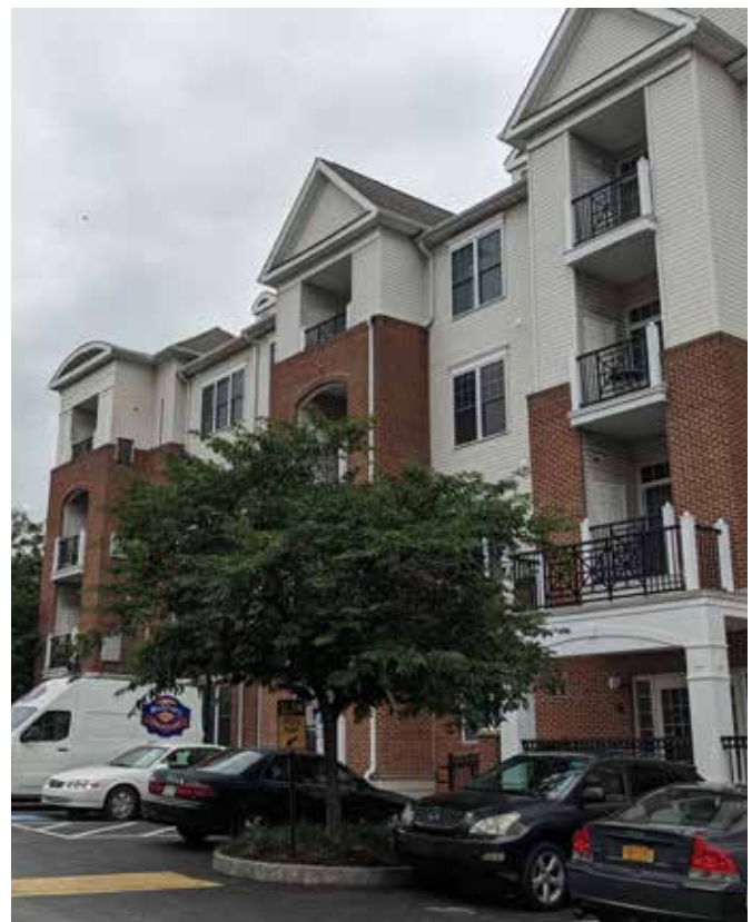
Surface parking is conveniently located along secondary building frontages internal to the site.
