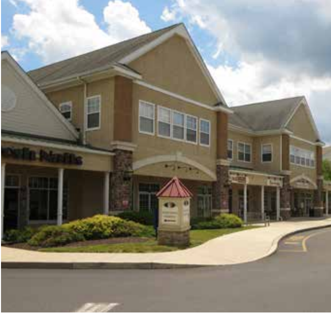
The commercial portion of the development includes a combination of 1- and 2-story buildings.
