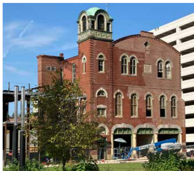
The SORA West development preserved the historic fire station building, which, when complete, will be reused as a brewpub and integrated into the overall design of the development.
