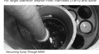
vaults complete sediment removal may be facilitated by removing a cartridge lid from an empty receptacle and inserting a jetting wand (not a vacuum wand) through the receptacle. Use the sprayer to rinse loosened sediment toward the vacuum hose in the MAW opening, being careful not to damage the receptacle.
