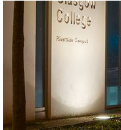
In-ground up lighting
