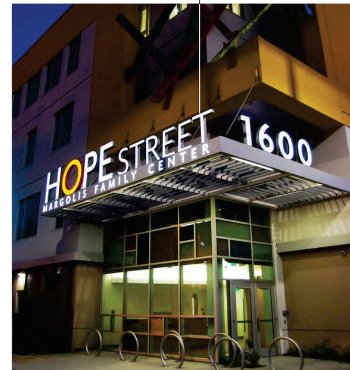
Face Illuminated Channel Letters Mounted on structural architectural rail
