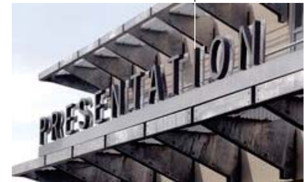
Halo Illuminated Channel Letters Mounted on structural architectural rail
