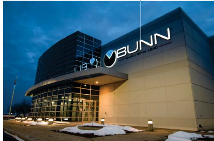
Face Illuminated Channel Letters Mounted to exterior EIFS wall panels
