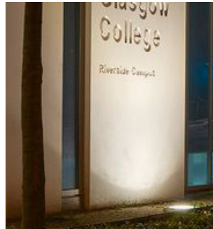
In-ground up lighting
