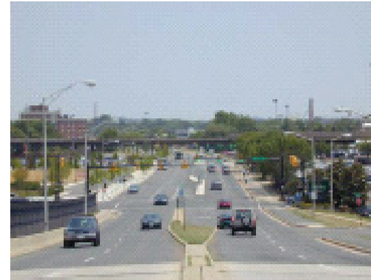
View of existing Eisenhower Avenue looking east
