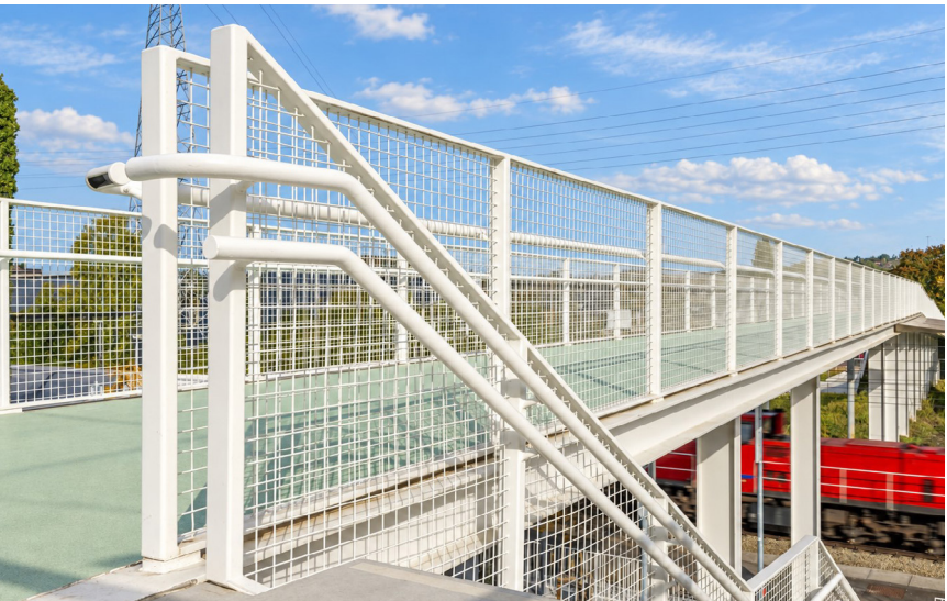
Pedestrian bridge detail
