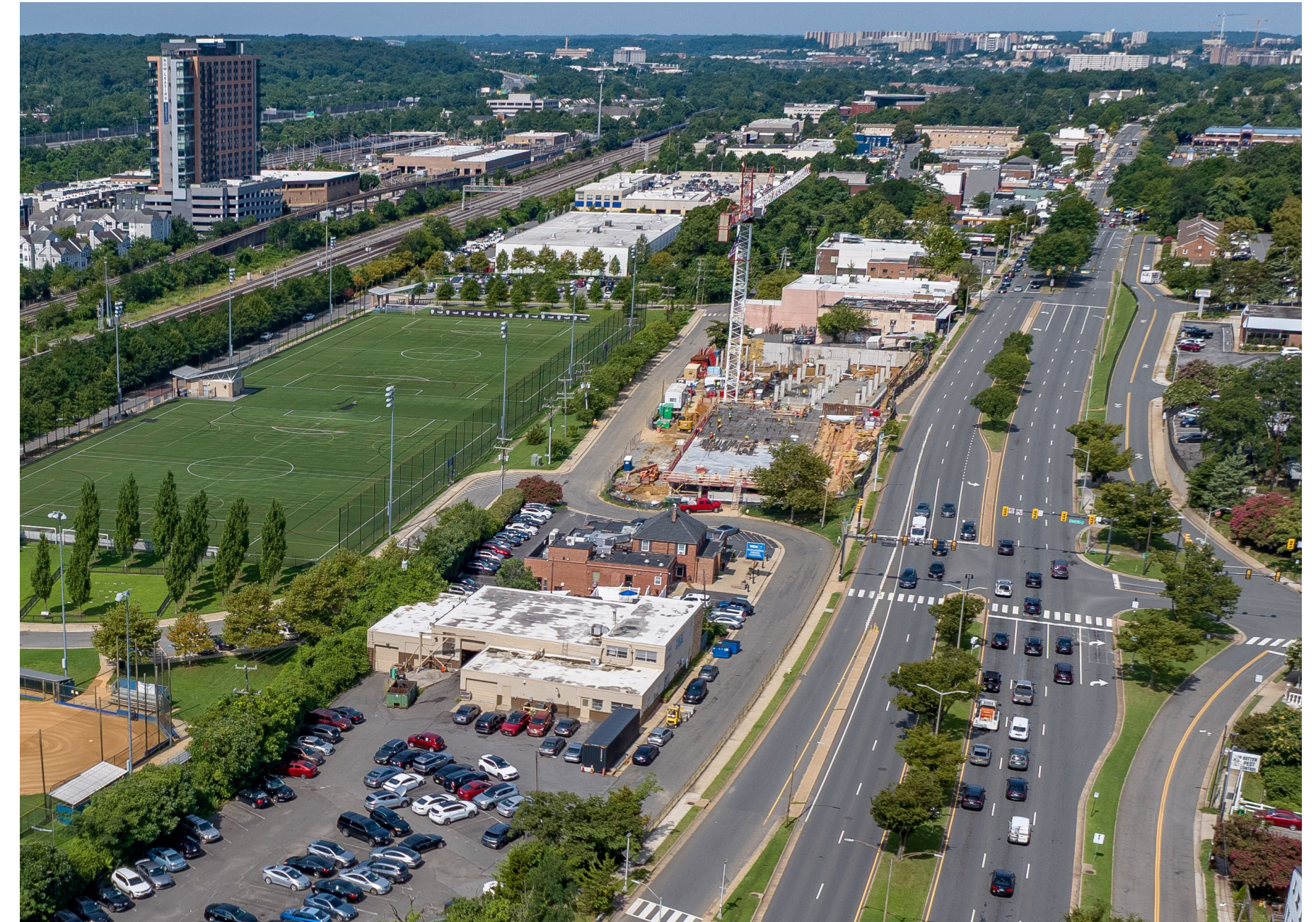
Aerial photo of Duke Street corridor, looking east, 2025
