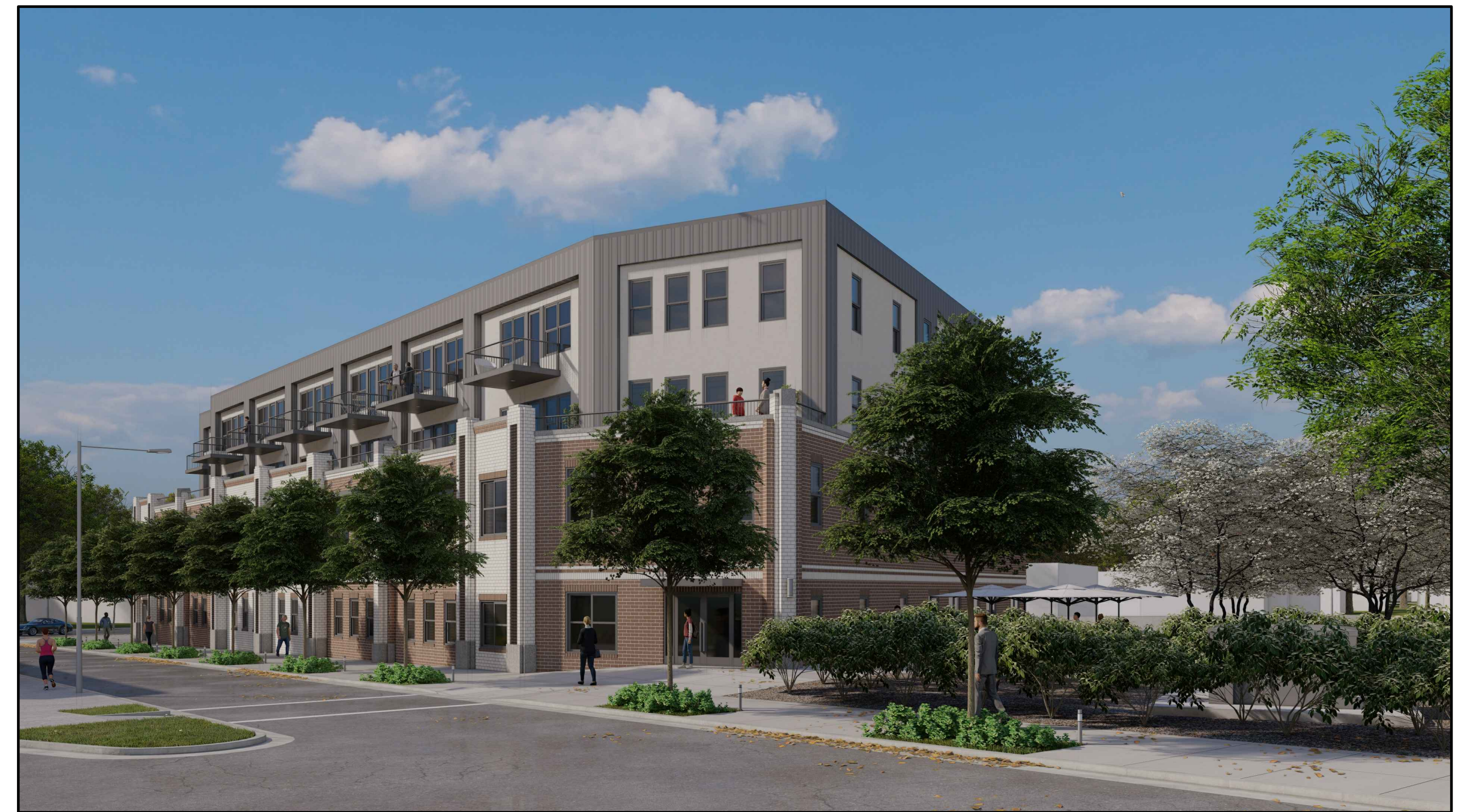
Facade Along Mt. Ida
