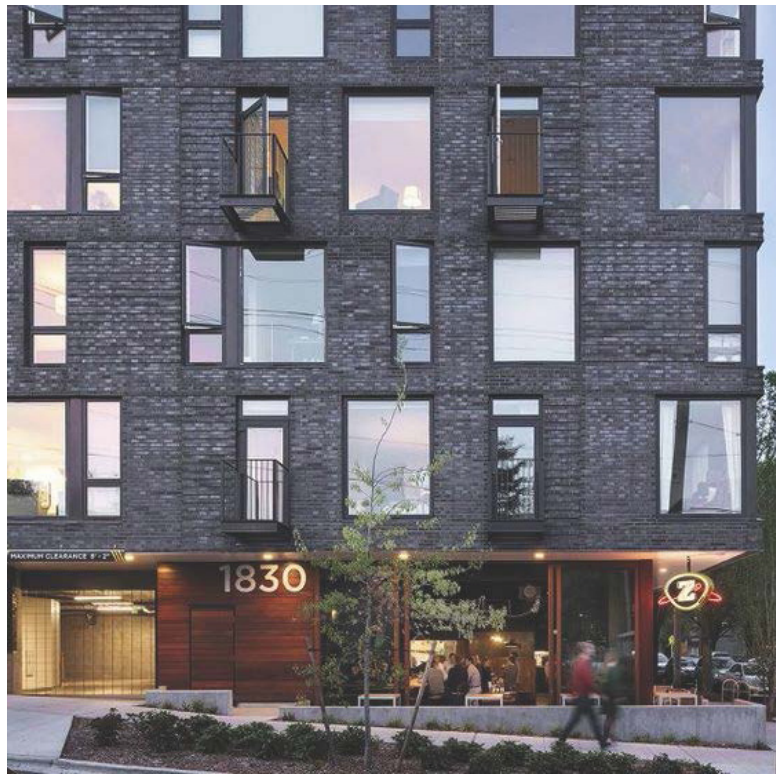
New development will encourage ground floor uses that enhance and activate the public realm.
