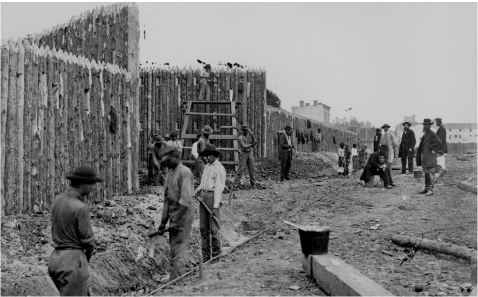
Barricades Being Constructed along Duke Street to protect the O&A Railroad from Confederate Cavalry (1861)
