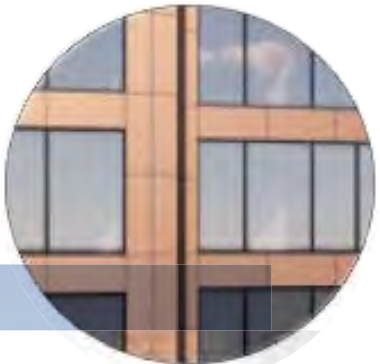
Road B Façade Window wall system with metal panel or Terracotta or Porcelain
