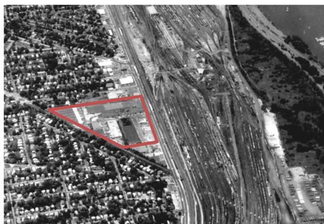
Figure 8. Detail from aerial photograph (1977) showing Potomac Yard (left) and Oakville Industrial Park (outlined in red) (Fairfax County, Virginia GIS).
