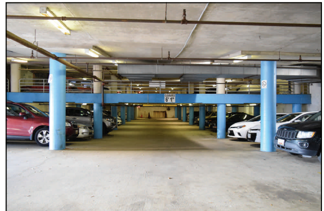
Figure 11. Photograph showing interior view of the lower parking level of the Solo Parking facility. (Image: RCG&A)
