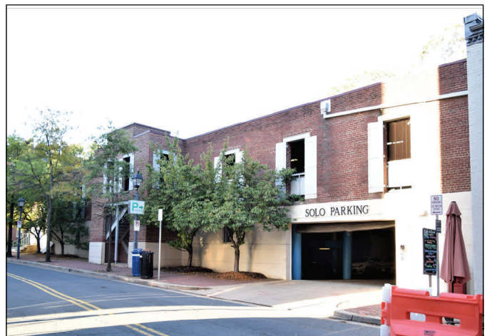
Figure 2. Photograph showing Solo Parking facility, 101 Duke Street, Alexandria, Virginia. (Image: RCG&A)
