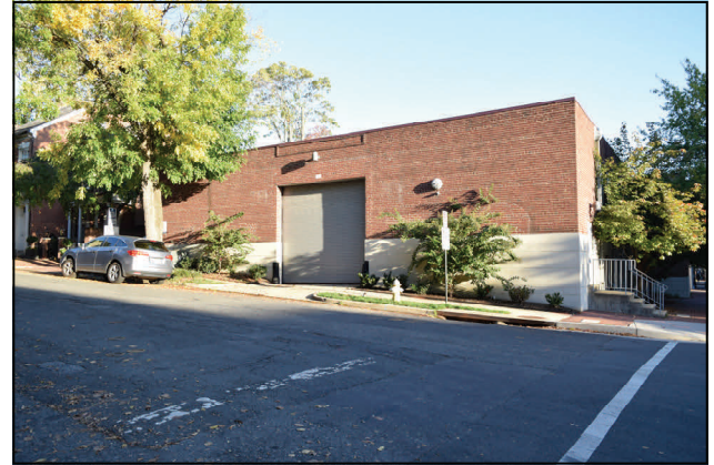
Figure 10. Photograph showing the southern elevation of the Solo Parking facility (Image: RCG&A).
