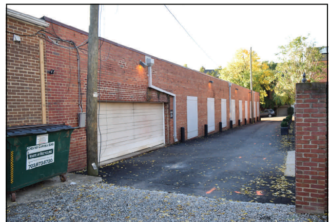
Figure 12. Photograph showing the entrance to the upper parking level of the Solo Parking facility, as accessed from the public alley (Image: RCG&A)
