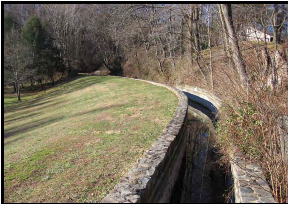
Figure 14. The (contemporary) reinforced headrace of Colvin Run Mill, which channels water eastward toward the mill from an impoundment of Colvin Run (Orientation west) (Photo: RCGA)
