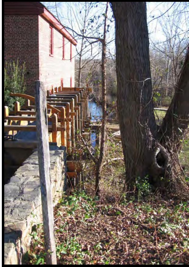
Figure 15. Junction of mill head race and wooden flume at Colvin Run Mill (orientation east). Note control gate at head of flume (left) and elevation of the race above the tailrace in the background (Photo; RCGA)
