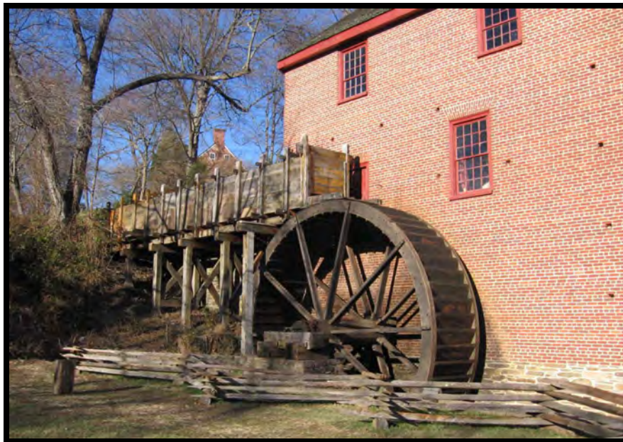
Figure 16. View of mill wheel and elevated wooden flume at Colvin Run Mill (orientation northwest) (Photo: RCGA)
