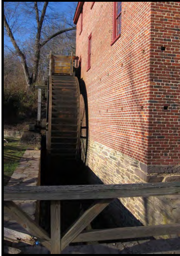
Figure 17. View of the exterior wheel-pit at Colvin Run Mill and the stone-reinforced upper portion of the mill's tail-race (RCGA)
