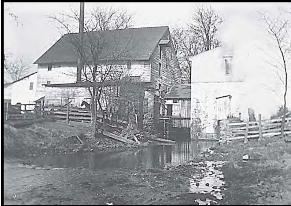
Figure 46. Post 1875 photograph of Hunt and Roberts' Cameron Mills (south façade), showing the addition that housed the steam engine and boiler installed in 1875-6 (Alexandria Library, Special Collections).
