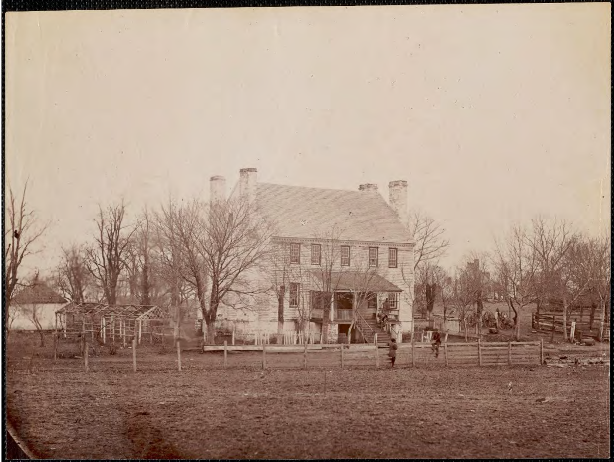
Figure 22. Grigsby House, Centreville, Virginia, Medford Historical Society & Museum, https://www.digitalcommonwealth.org/search/commonwealth:h128s849z , note the bars over the basement windows.
