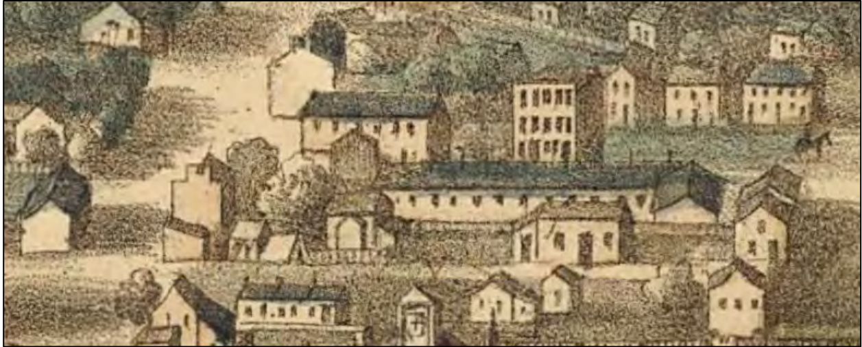
Figure 36. Detail of Magnus' "Birds eye view of Alexandria, Va., 1863. View is facing west. Duke Street is running vertically along the left side of the image here, Commerce Street is running diagonally at the top right, Fayette Street is running horizontally at the bottom, Payne Street is running horizontally in the middle, and West Street is running horizontally at the top. Visible here are the long "Contraband" barracks along Payne Street (center), 1207 Duke Street (far left, but on the right [north] side of Duke Street)), and 1315 Duke Street (top left)
