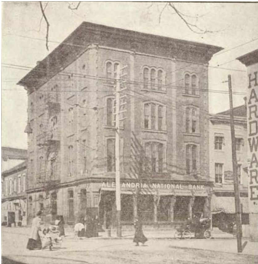
Figure 16 Alexandria National Bank Building, 325 King Street, corner of N. Royal, from Alex. J. Wedderburn, Souvenir Virginia Tercentennial of Historic Alexandria, Va., Past and Present (Alexandria, 1907). Originally built by Daniel T. Witmer in 1859 and known as The Witmer Building.
