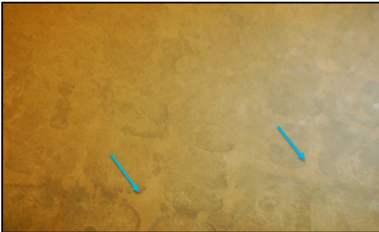
Figure 4. Silt covering geogrid material on 26 May 2022 (blue arrows indicating to exposed geogrid material).
