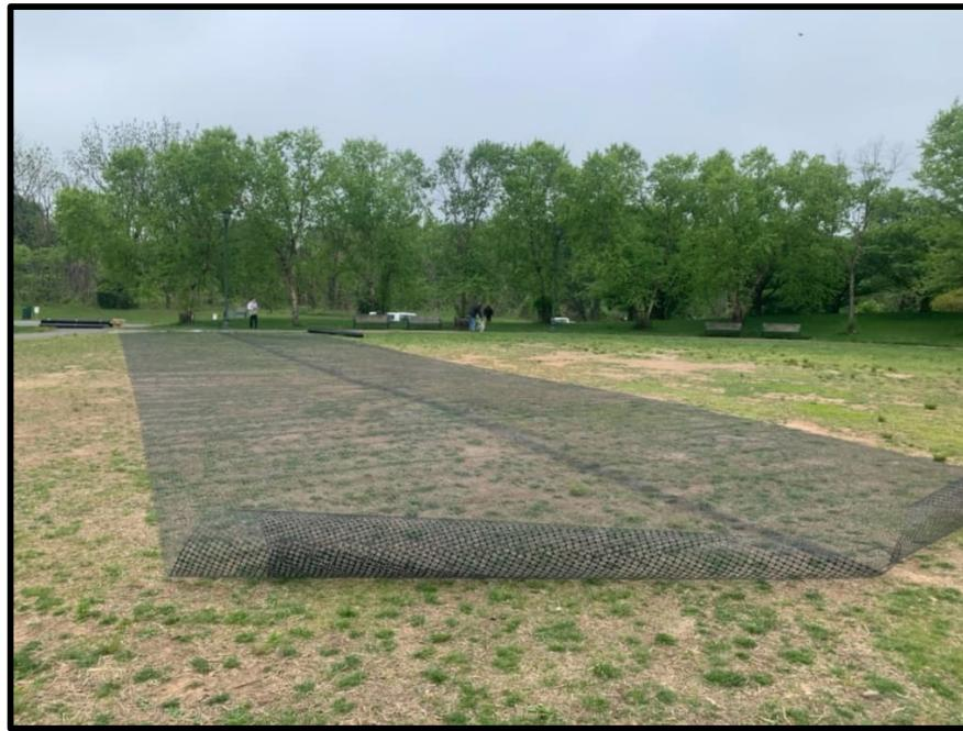
**Figure 2. Assembled geogrid material used to prepare Ben Brenman Pond bottom.**
