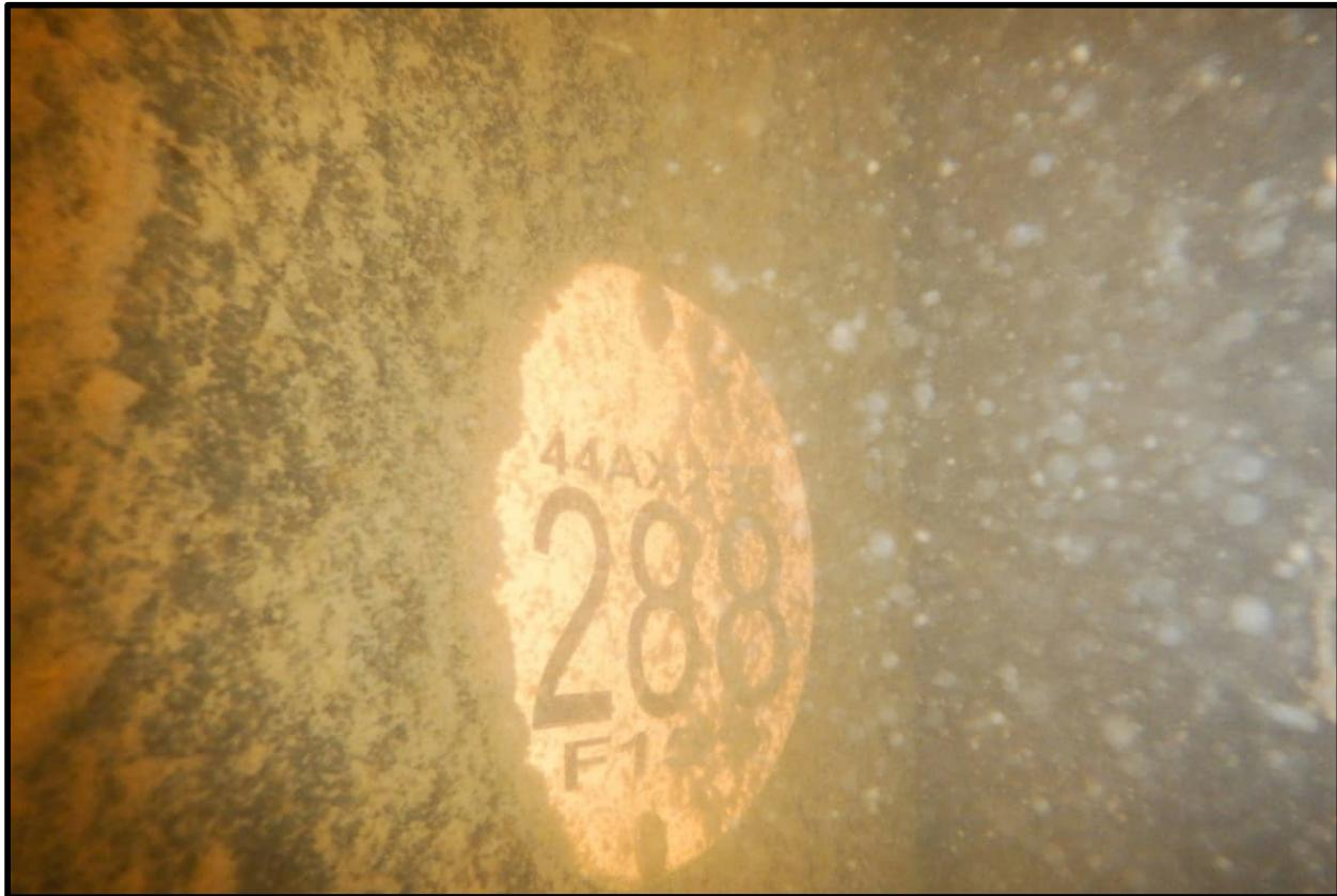
Figure 5. Silt covering outer fabric on timber bundles on 26 May 2022.
